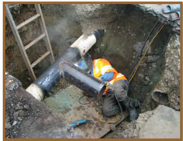
Image 3-4: District Staff Welds a Pipe Repair (Potential Ignition Source)
