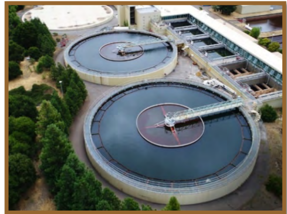
Image 3-7: San Geronimo Water Treatment Plant (Aboveground Asset)
