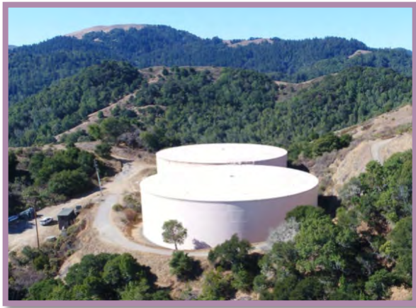
Image 2-3: District Tanks in the Wildland Urban Interface (WUI)
