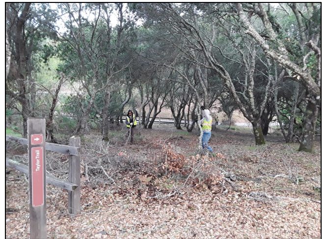
Photo 23: Taylor Trail Fuelbreak Construction.
