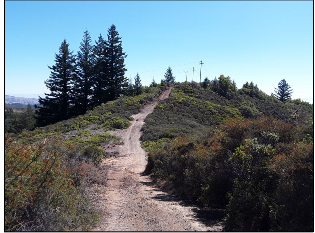
Photo 5: PG&E Veg Maintenance Coordination on Access Road leading to Pole Structure.
