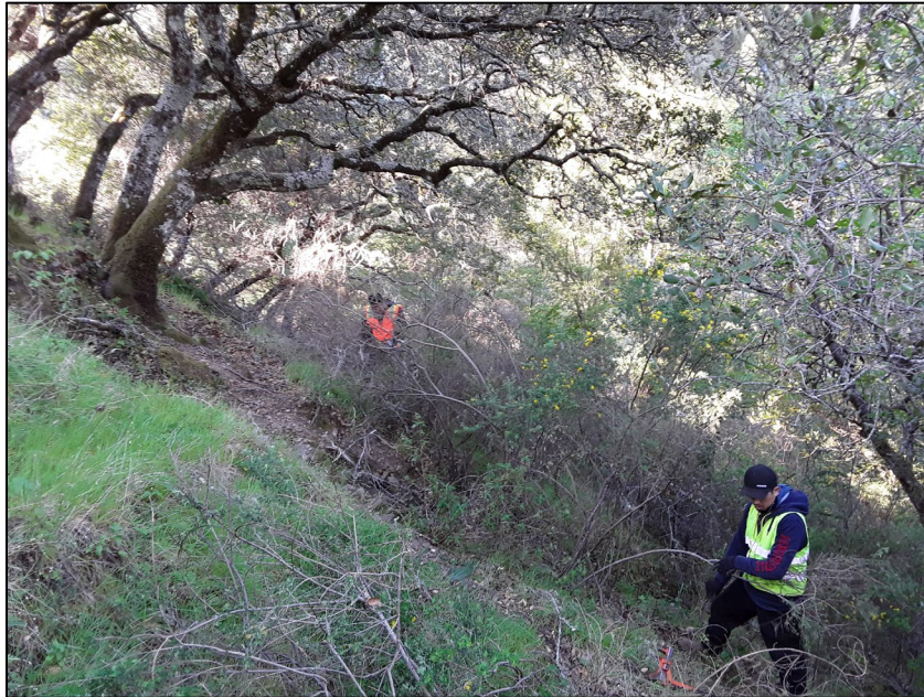
Photo 18: Broom Maintenance at Indian Crown Fuelbreak
