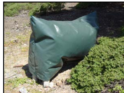
INSULATED BLANKET ENCLOSURE (SECURITY/FREEZE)
