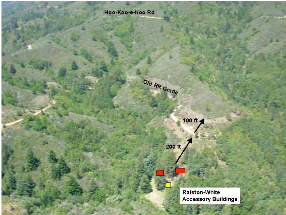
Figure 5 Example of Fuelbreak Constructed at end of W. Blithedale Canyon
