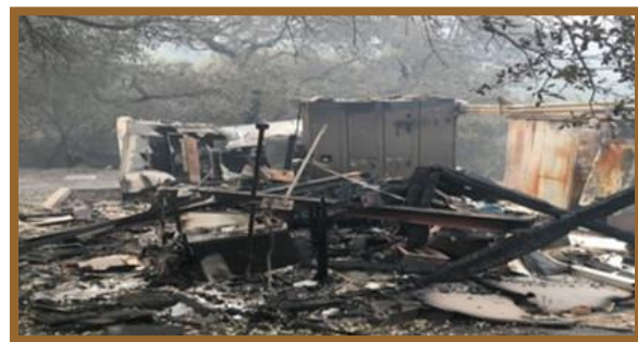
Image 3-2: City of Napa Pump Station Near Silverado Country Club Destroyed During the 2017 Atlas Fire (Direct Hazard) 4
