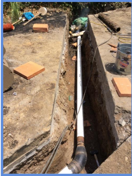
Image 5-1: Upsizing Water Main for Improved Fire Flow
