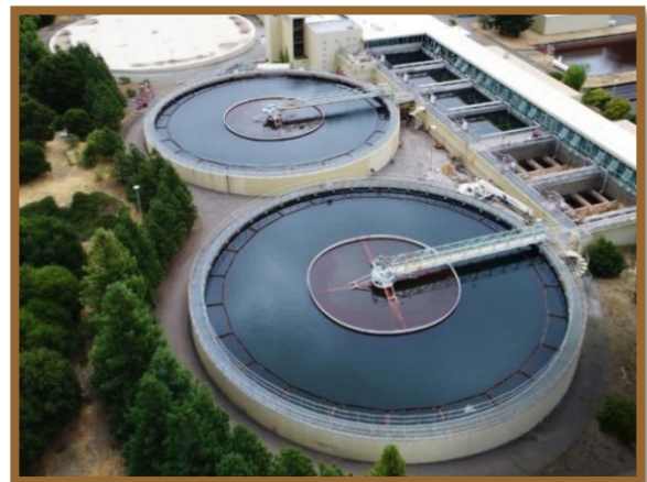
Image 3-7: San Geronimo Water Treatment Plant (Aboveground Asset)
