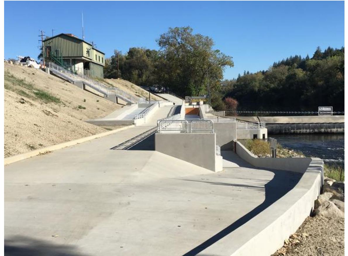
Russian River Collectors, Diversion Dam, and Fish Passage
