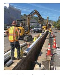
A 2022 pipeline replacement project on Third Street in San Rafael replaced 6,570-feet of 95-year-old cast iron pipe with new welded steel pipe. The proposed rate adjustment will increase the amount of aging pipeline Marin Water is able to replace per year.
