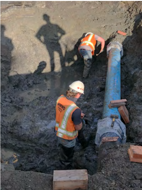
Marin Water Operations staff perform emergency underground pipeline repairs.
