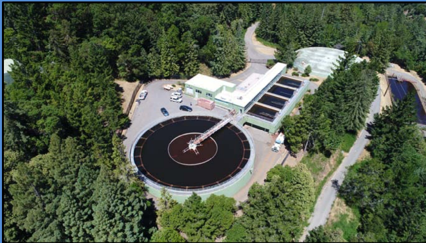
Bon Tempe Treatment Plant
