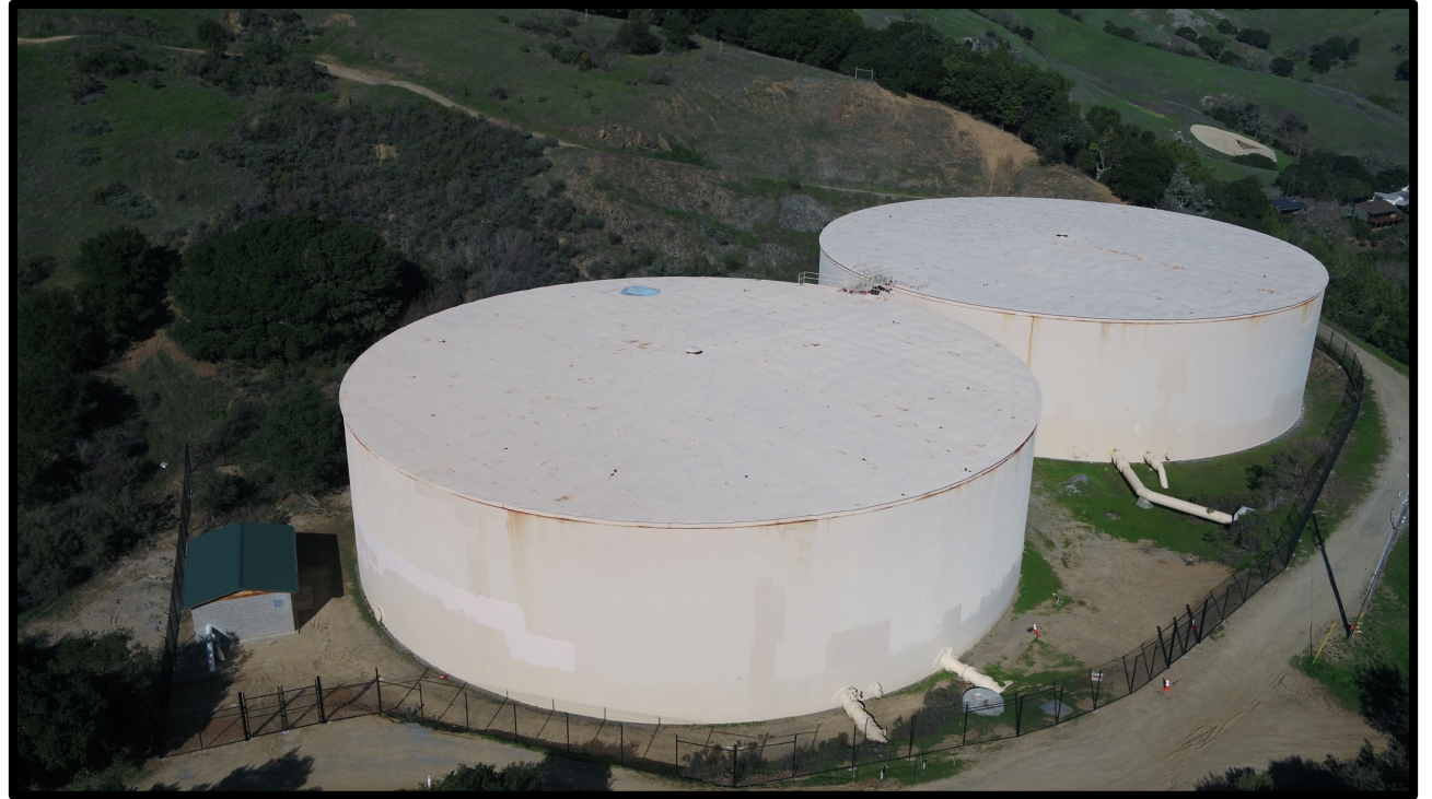
Smith Saddle Storage Tanks Provide 10 MG of Storage
