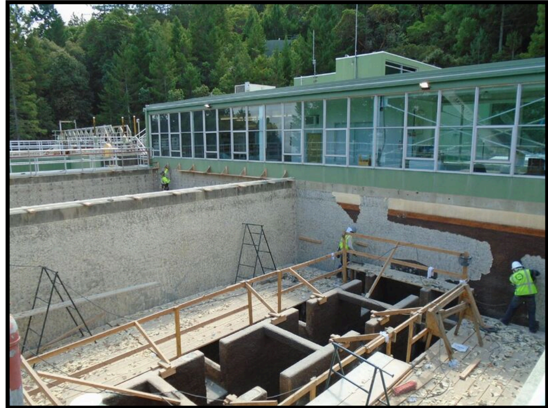
Seismically upgrading filters at Bon Tempe Treatment Plant (2017)
