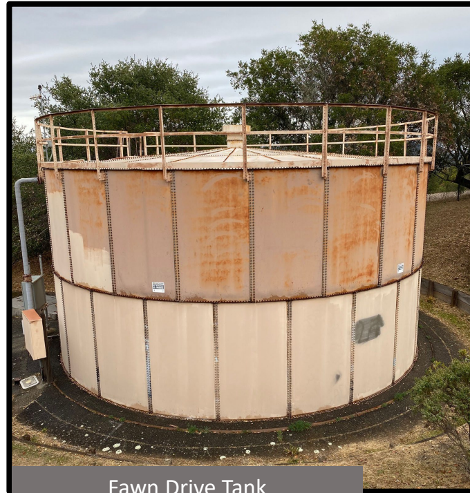
Fawn Drive Tank Bolted steel tank, installed 1985
