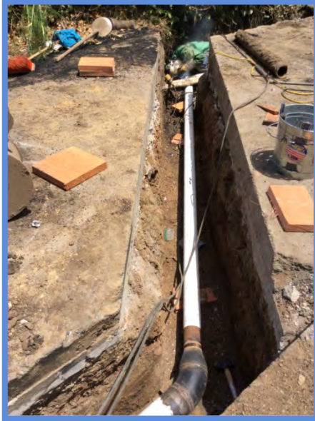
Image 5-1: Upsizing Water Main for Improved Fire Flow
