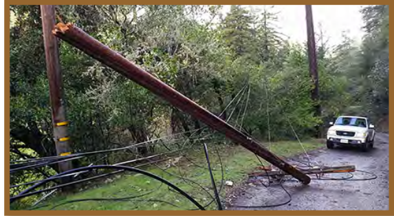
Image 3-1: Downed Power Lines Near Kent Lake (Ignition Source)
