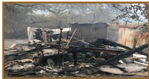
Image 3-2: City of Napa Pump Station Near Silverado Country Club Destroyed During the 2017 Atlas Fire (Direct Hazard) 4
