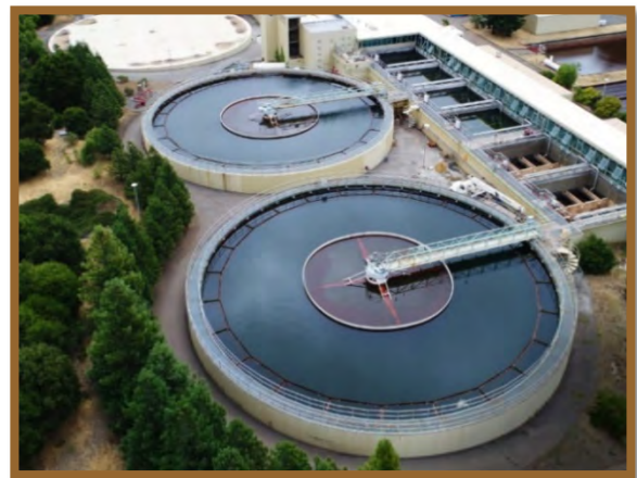
Image 3-7: San Geronimo Water Treatment Plant (Aboveground Asset)
