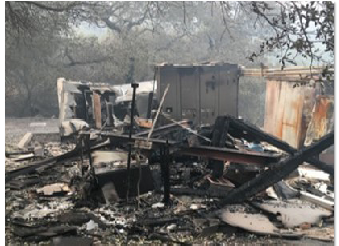
City of Napa Pump Station Destroyed During 2017 Atlas Fire
