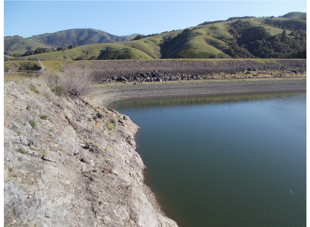
Soulajule Reservoir and Dam
