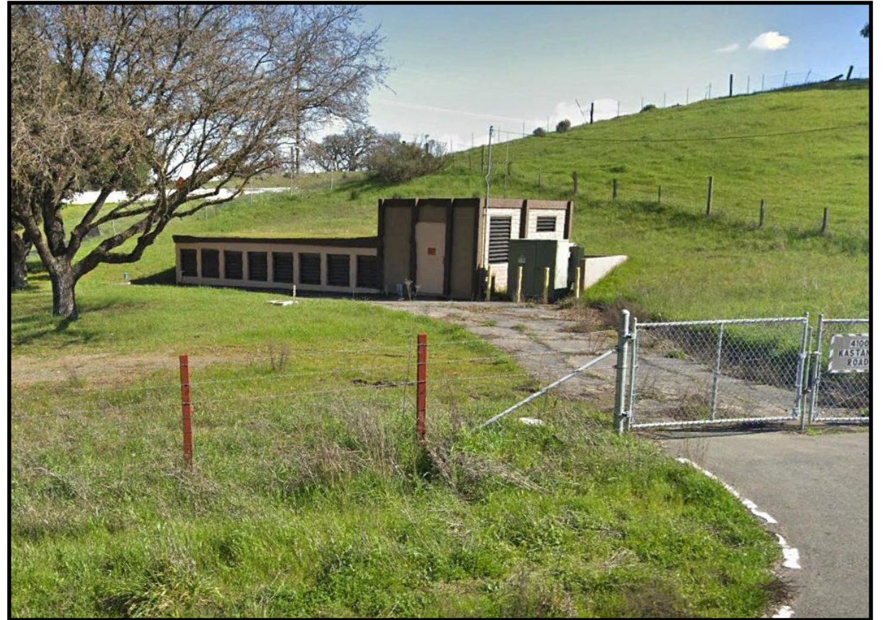
Kastania Pump Station, Kastania Rd, Petaluma
