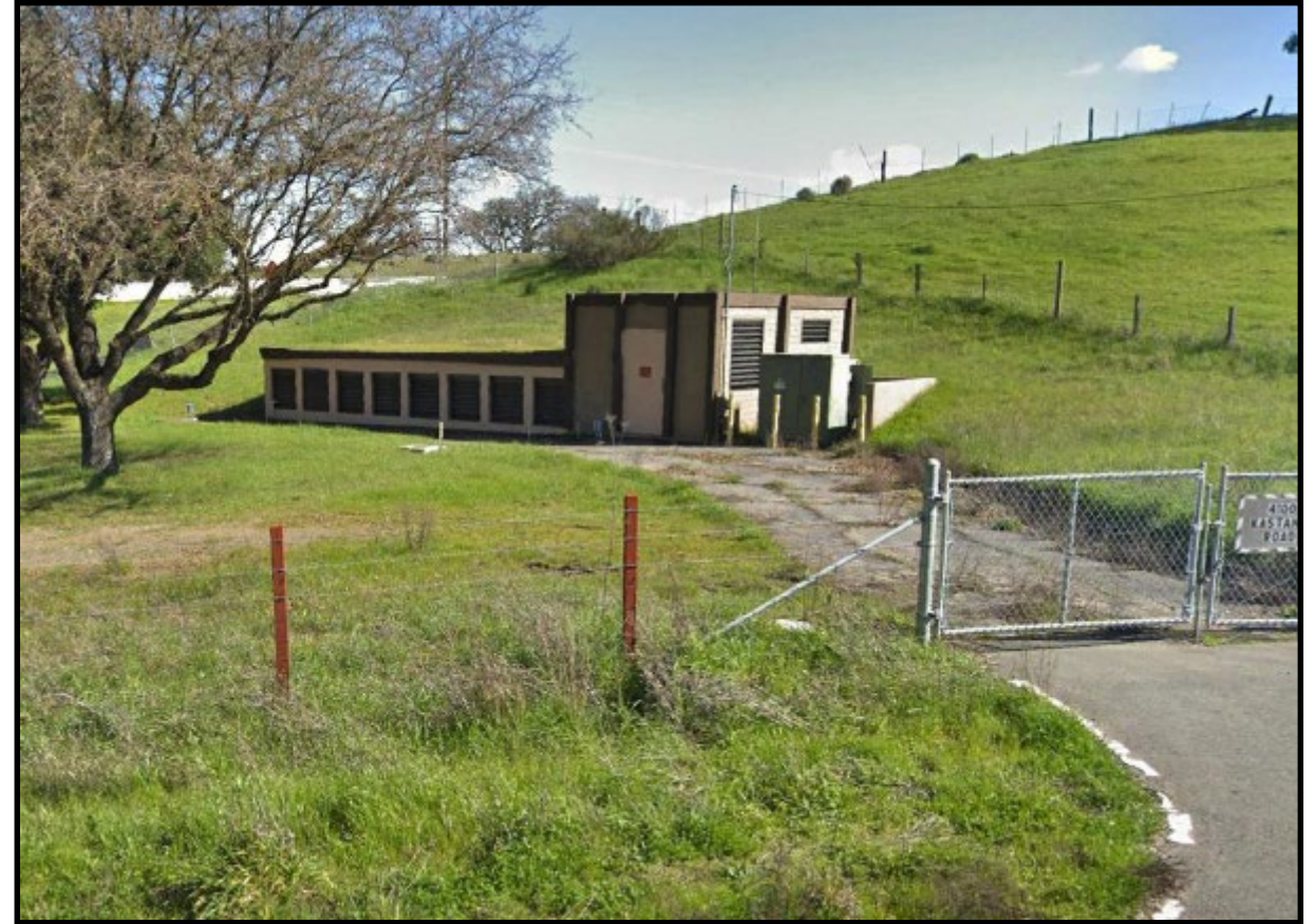
Kastania Pump Station, Kastania Rd, Petaluma
