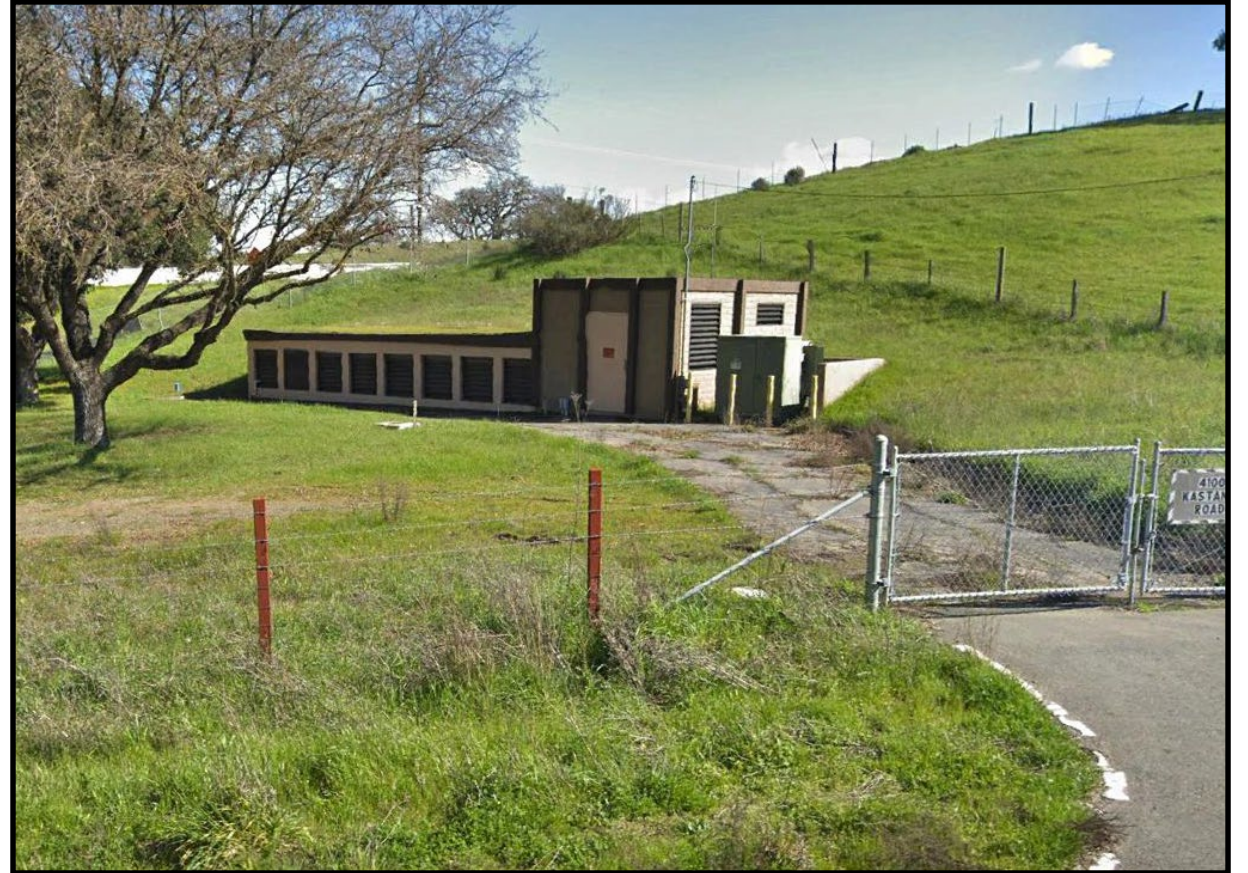
Kastania Pump Station, Kastania Rd, Petaluma
