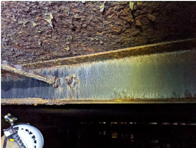
Photo 4-5 intact coating on web
