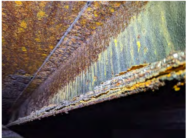
Photo 4-24 Moderate corrosion on flange
