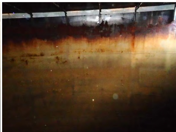
Photo 4-31 Corrosion on shell above waterline
