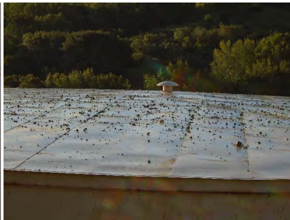
Photo 4-46 rock debris on roof
