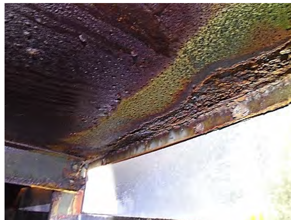
Photo 4-7 Coating and corrosion above shell vents and roof plates
