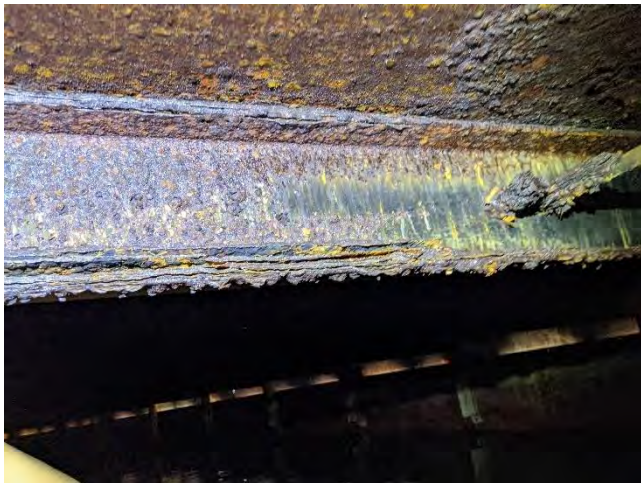
Photo 4-23 Moderate corrosion on flange
