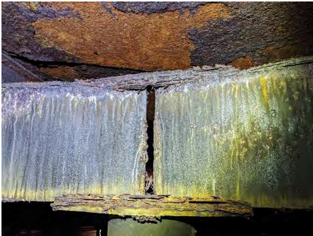
Photo 4-17 Failed coating moderate corrosion
