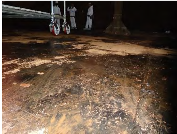
Photo 4-33 Blisters and fractures on floor
