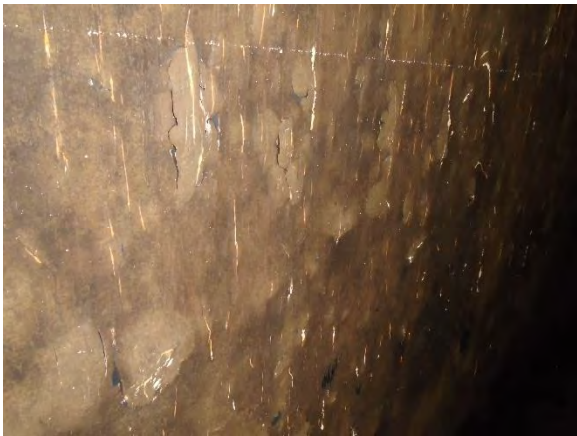
Photo 4-28 Blisters and fractures
