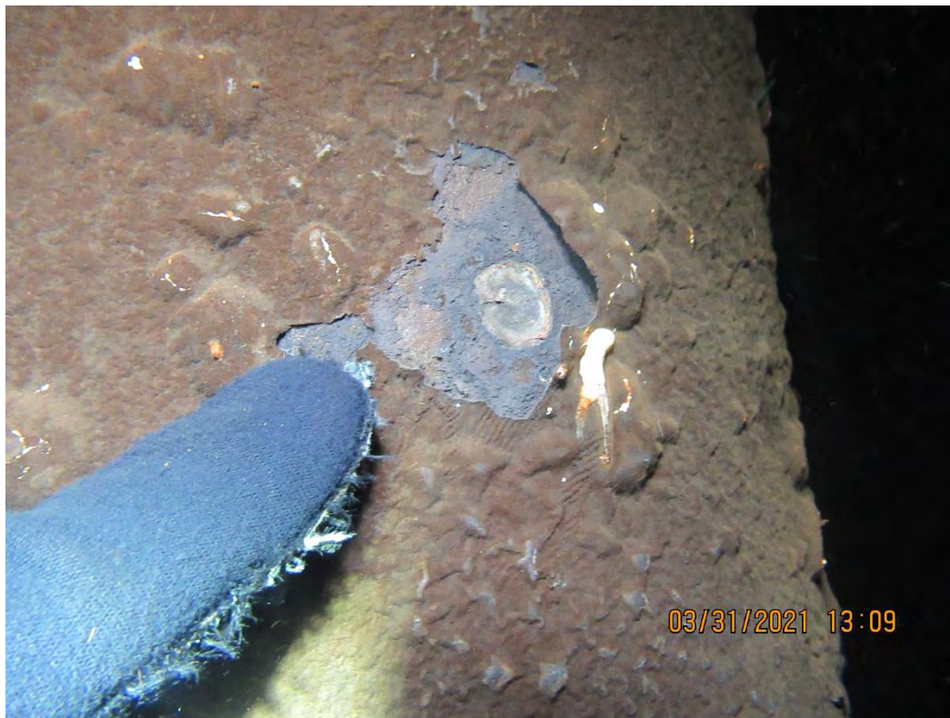
Image 22 – Exposed steel beneath a popped column coating blister
