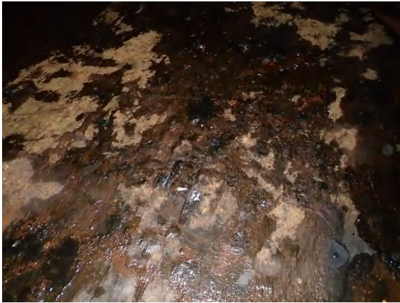
Photo 4-32 Blisters and fractures on floor
