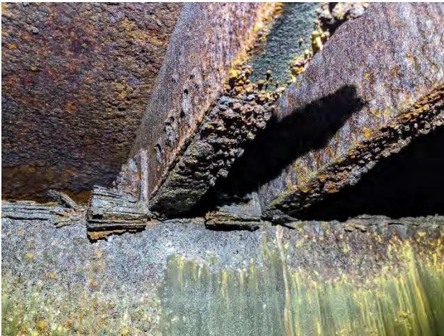
Photo 4-15 Moderate corrosion on connections
