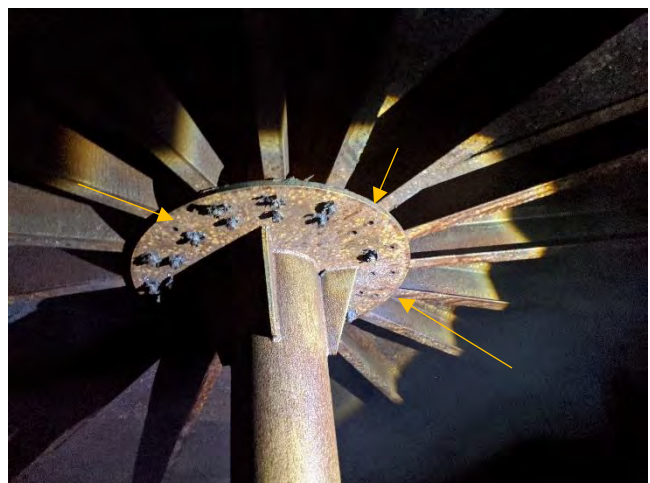
Photo 4-37 missing bolts
