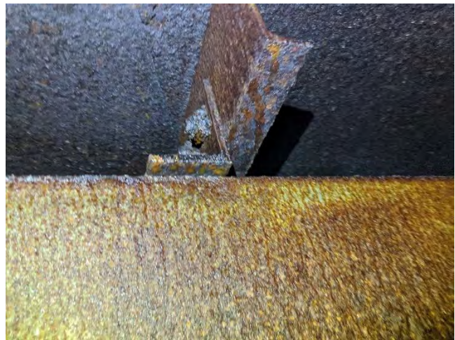
Photo 4-35 failed coating & minor corrosion
