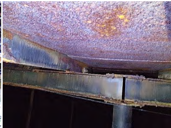
Photo 4-12 Failed coating on supports and roof plates
