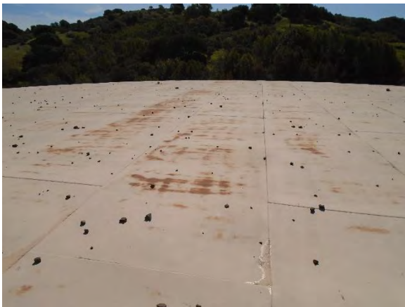
Photo 4-39 Corrosion developing through coating
