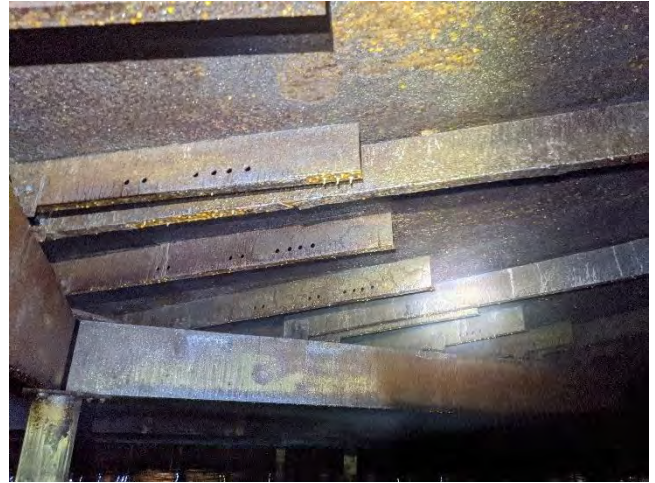
Photo 4-29 minor corrosion
