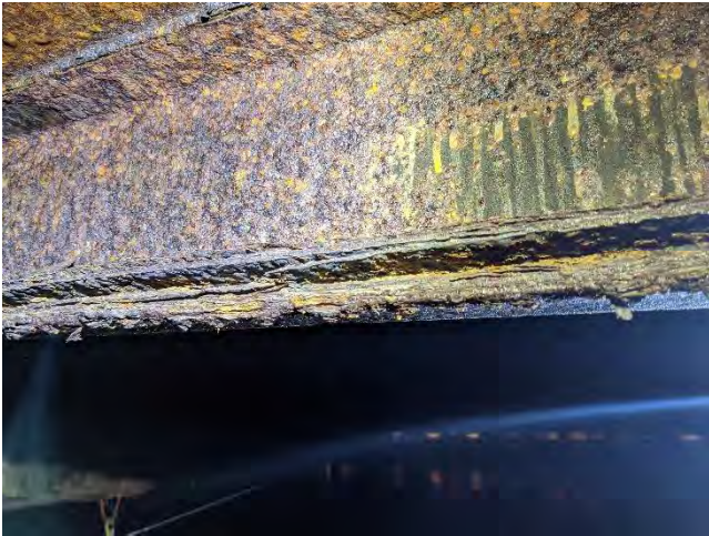
Photo 4-21 Moderate corrosion on flange
