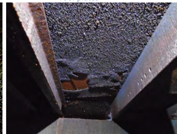
Photo 4-26 Failed coating on roof plates
