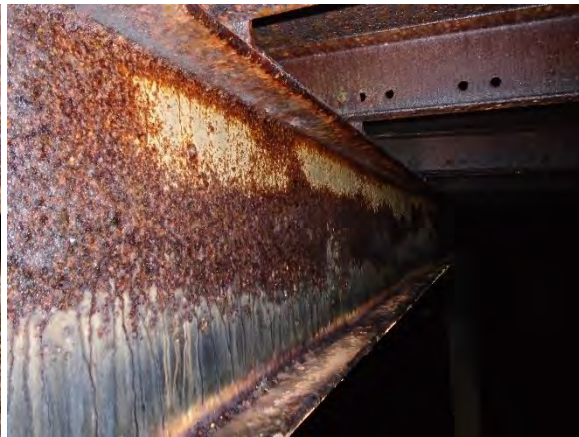
Photo 4-18 Failed coating center bay
