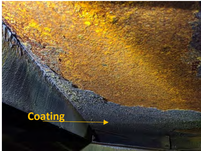
Photo 4-9 bare steel and failed coating
