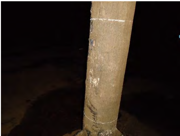
Photo 4-34 Blisters and fractures on column
