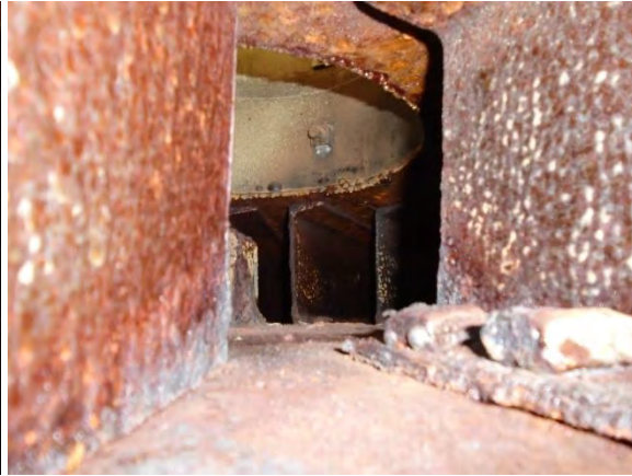
Photo 4-22 Rafter ends above dollar plate
