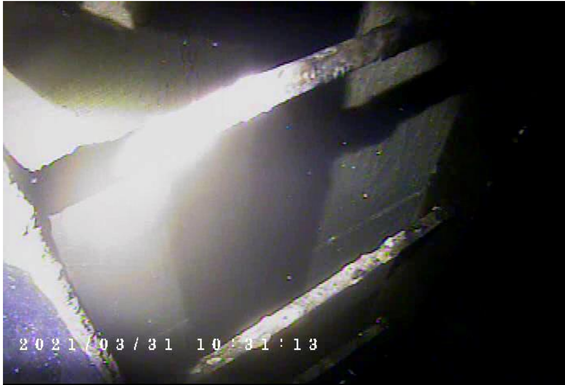
Image 1 – Minor pitting on ladder coating
