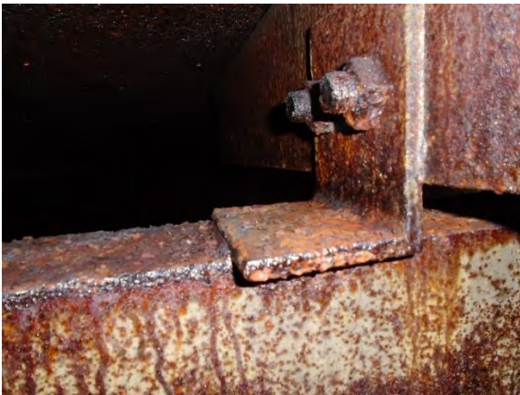
Photo 4-17 Failed coating center bay
