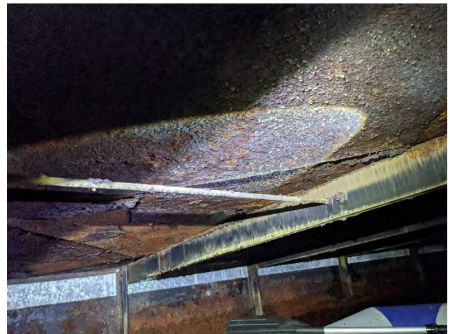
Photo 4-2. Metal loss on rafter/outer bay
