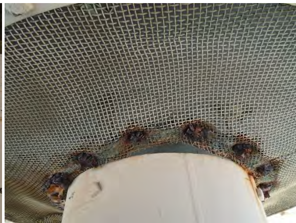
Photo 4-42 Bolt corrosion. No bug screen
