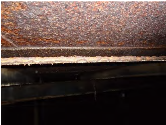
Photo 4-13 Failed coating roof plates / INT bay
