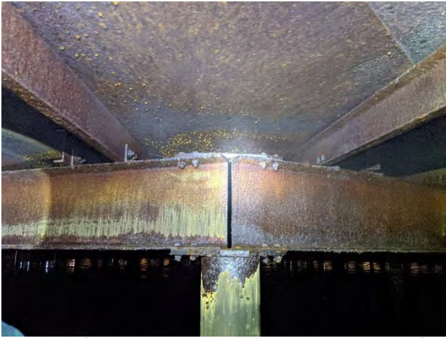
Photo 4-26 minor corrosion on center girder
