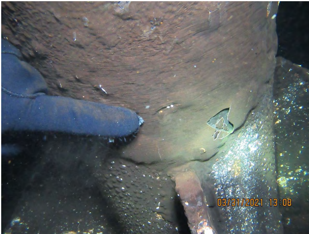
Image 20 – Typical blistering at the base of a column
