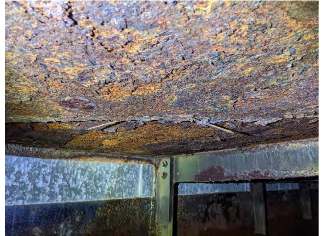
Photo 4-4. Moderate corrosion on roof plate
