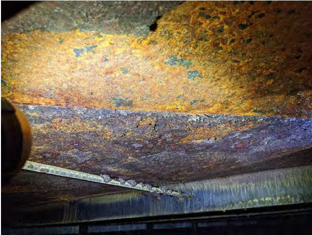
Photo 4-3. Failed coating on roof plate
