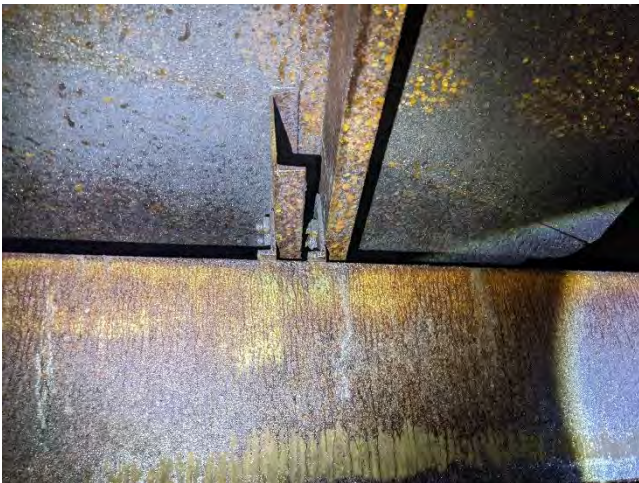
Photo 4-34 failed coating & minor corrosion
