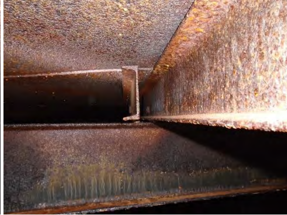
Photo 4-16 Failed coating/INT bay
