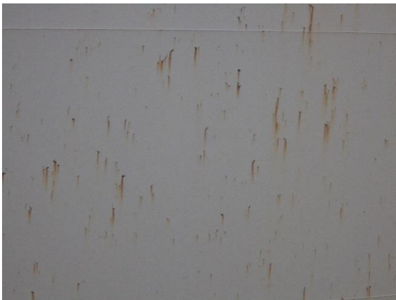
Photo 4-45 Rock damage on shell
