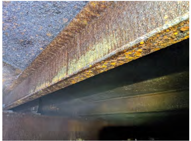
Photo 4-27 minor corrosion
