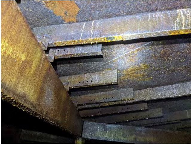
Photo 4-28 minor corrosion
