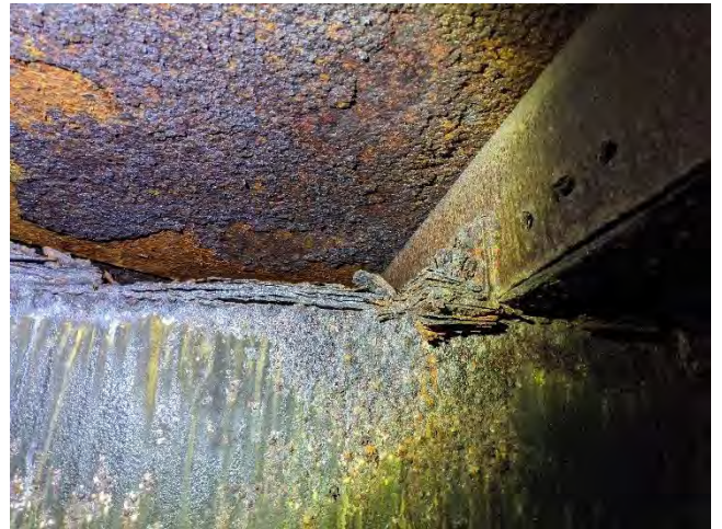
Photo 4-16 moderate corrosion
