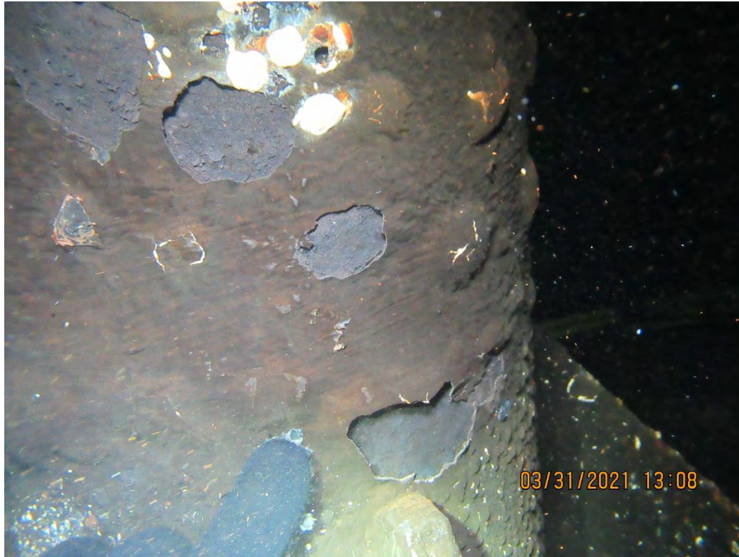
Image 21 – Multiple popped blisters at the base of a column
