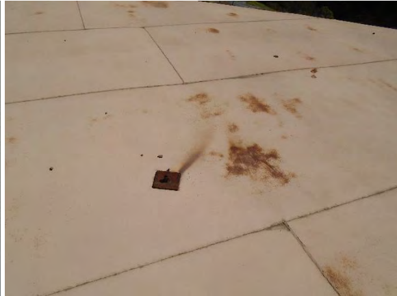
Photo 4-38 Carbon steel anode covers
