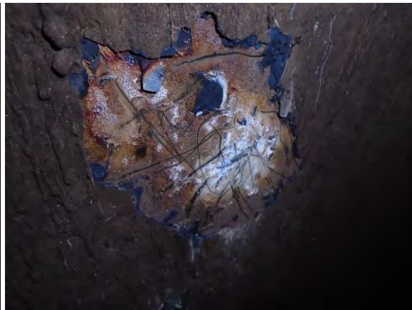
Photo 4-29 Steel being protected by C/P
