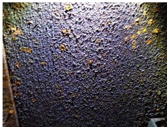
Photo 4-25 Failed coating on roof plates
