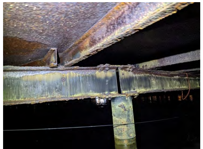
Photo 4-20 Failed coating intermediate bay
