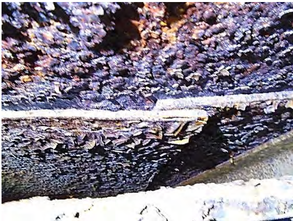
Photo 4-11 Failed coating and corrosion on plate overlaps
