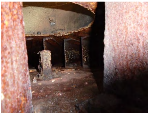
Photo 4-23 Rafter ends above dollar plate
