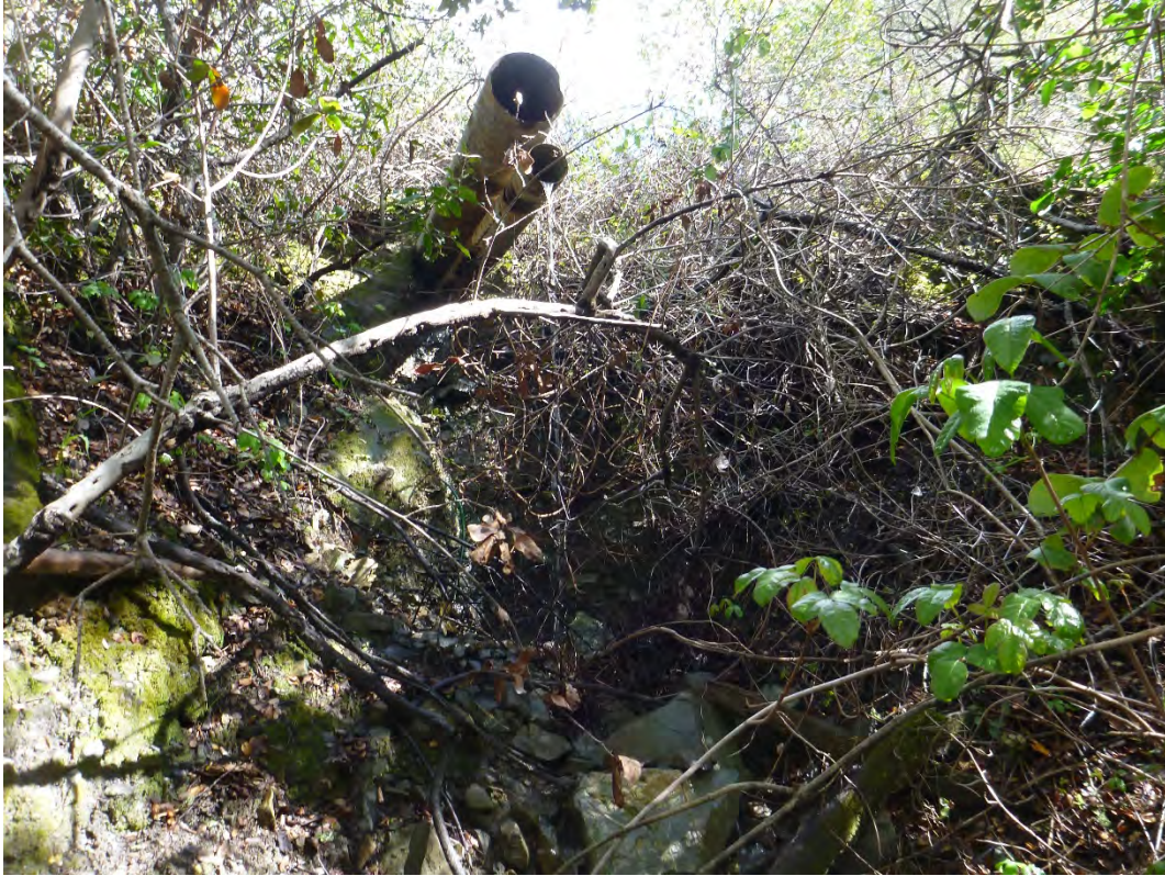
Drain pipes emanating from fill slope at west end of site. Note water draining from lower pipe. Photo by GEI.
