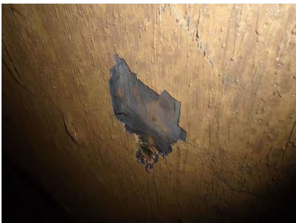
Photo 4-30 Under blister steel being protected
