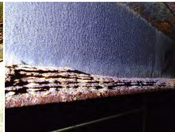
Photo 4-8 Failed coating and corrosion on rafter
