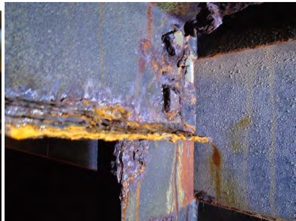
Photo 4-2. Metal loss on rafter/outer bay
