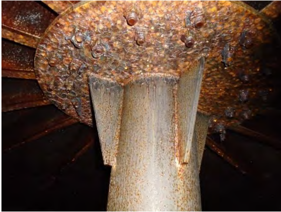
Photo 4-21 Failed coating on dollar plate
