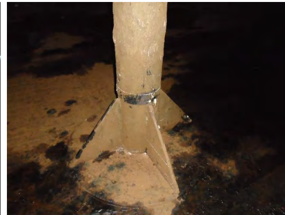
Photo 4-35 Blisters and fractures on column base
