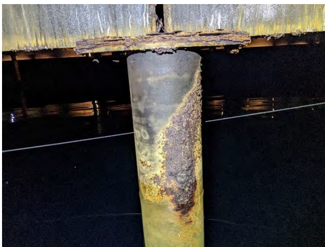
Photo 4-19 Failed coating on support column
