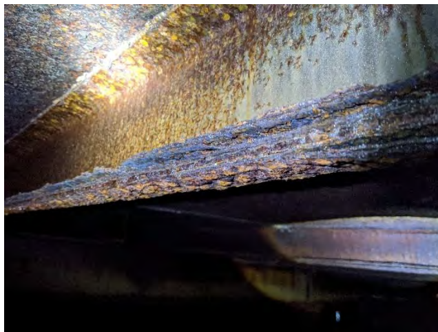
Photo 4-25 Moderate corrosion on flange
