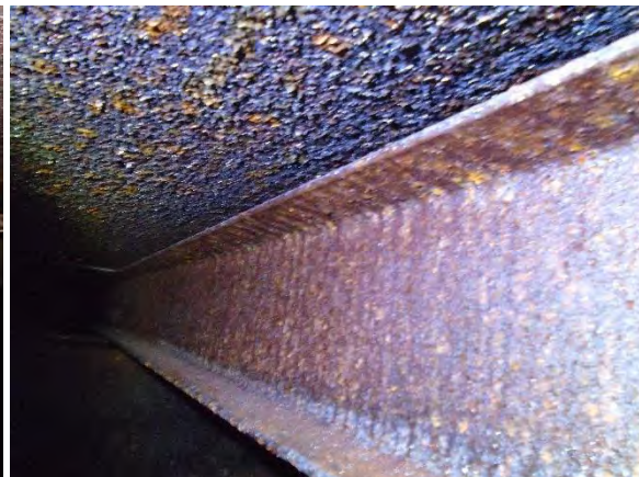
Photo 4-14 Failed coating / INT Bay
