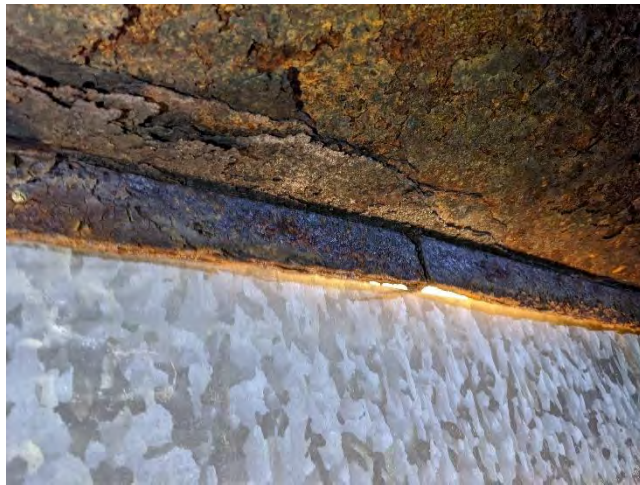
Photo 4-11 Gaps between sheet metal
