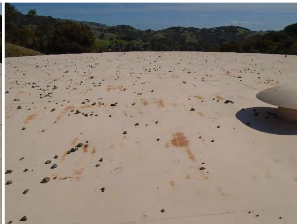
Photo 4-40 Corrosion developing through coating
