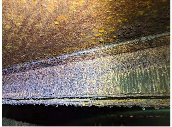
Photo 4-22 Moderate corrosion on flange
