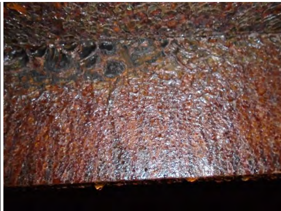
Photo 4-20 Center bay rafters fused to roof plate
