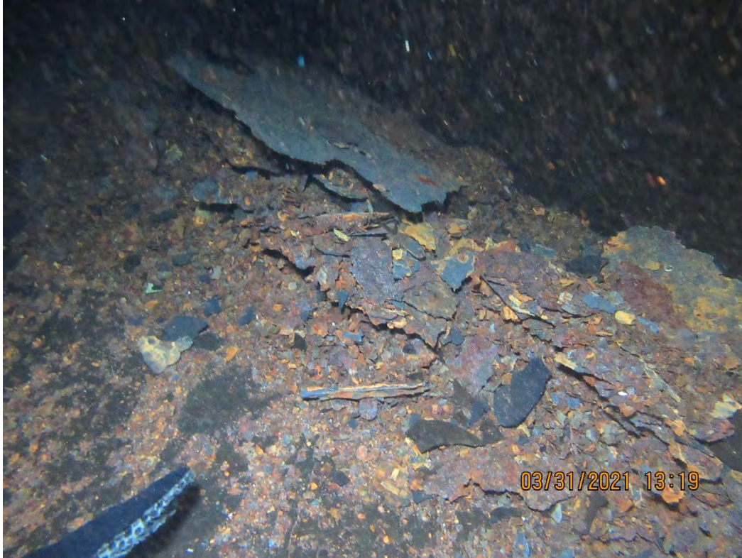
Image 9 – Rust pile on floor at wall in northeast quadrant
