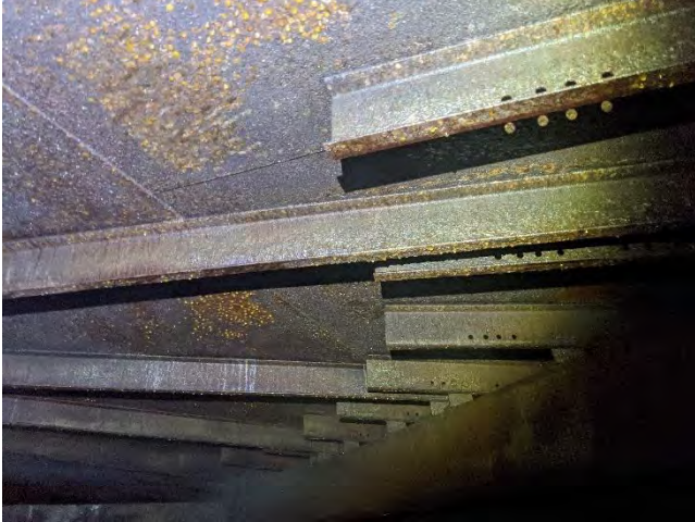
Photo 4-32 failed coating & minor corrosion
