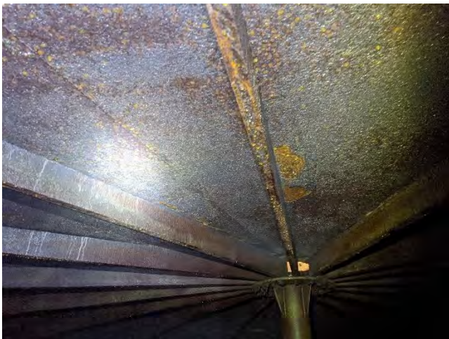
Photo 4-30 failed coating & minor corrosion
