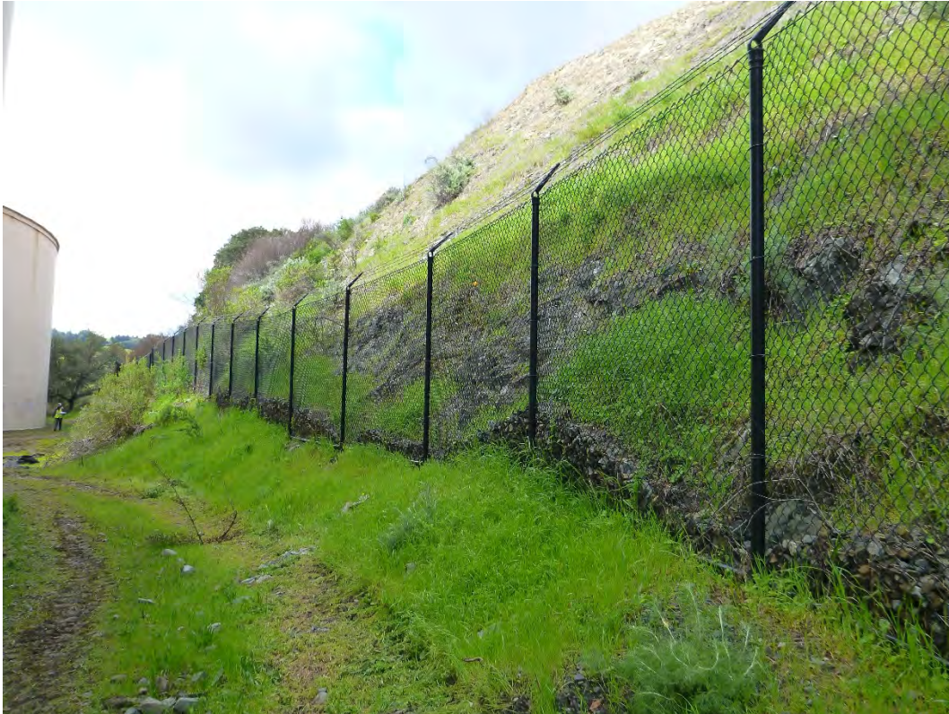
Perimeter fencing along northwest side of tanks. Note rock debris piled against base of fence. Photo by GEI.
