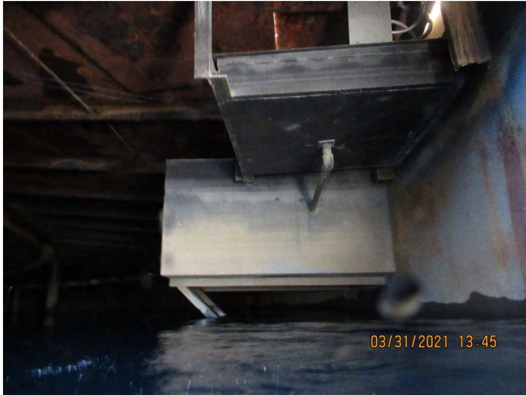
Image 3 – Weir box/overflow
