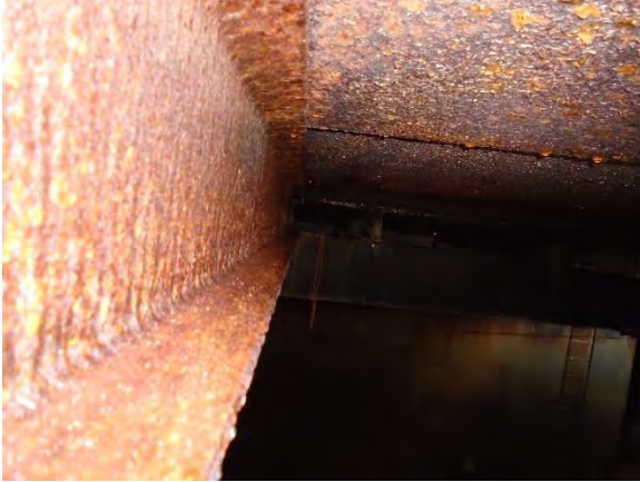
Photo 4-15 Failed coating/ INT bay
