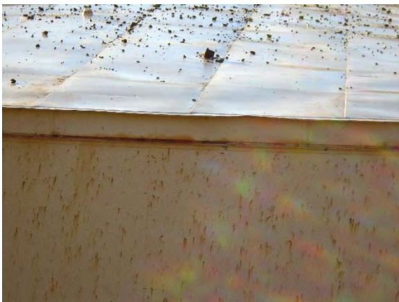
Photo 4-47 Rock damage on shell
