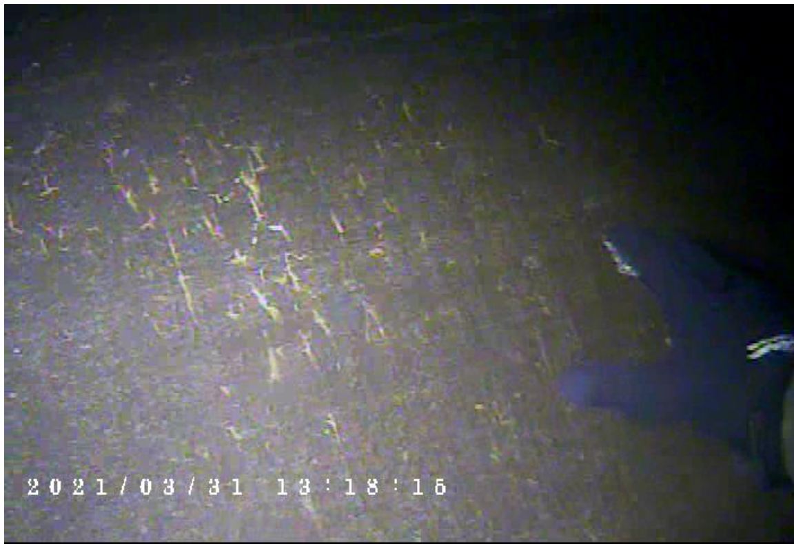
Image 6 – 2-foot-wide area of cracking paint 10-feet left of the ladder (typical)
