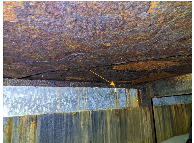
Photo 4-12 holes found in sheet metal
