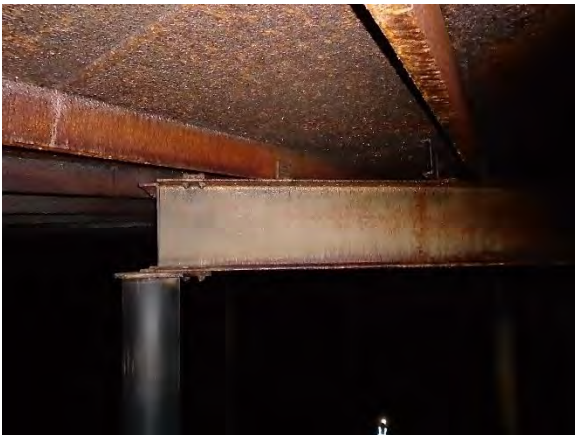
Photo 4-19 Center bay failed coating
