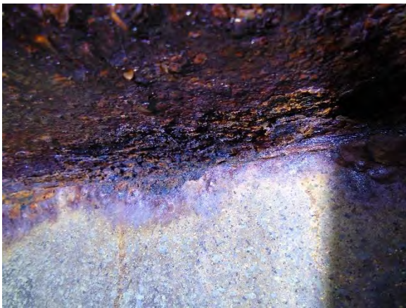
Photo 4-5 Rafter fused to roof plate
