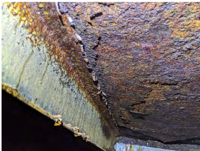
Photo 4-13 Moderate corrosion on flange
