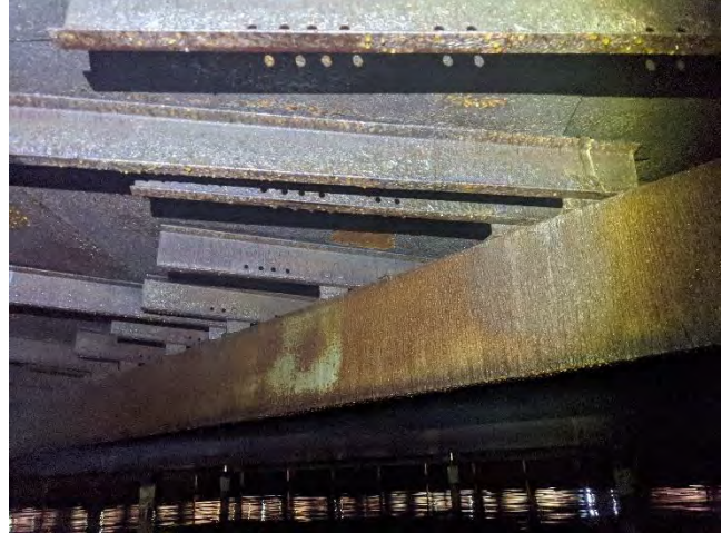
Photo 4-33 failed coating & minor corrosion
