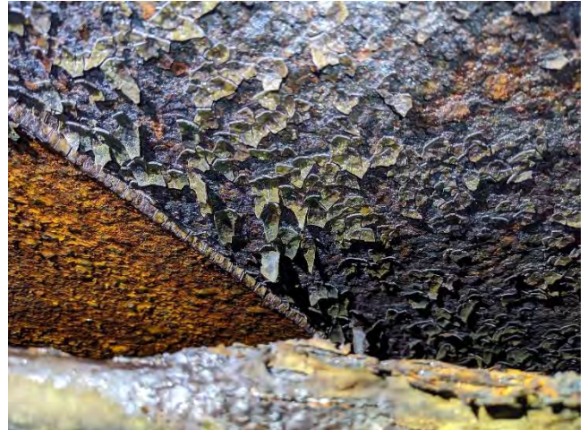
Photo 4-10 failed coating
