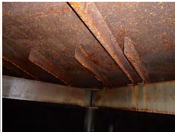
Photo 4-24 Failed coating on rafters and roof plates
