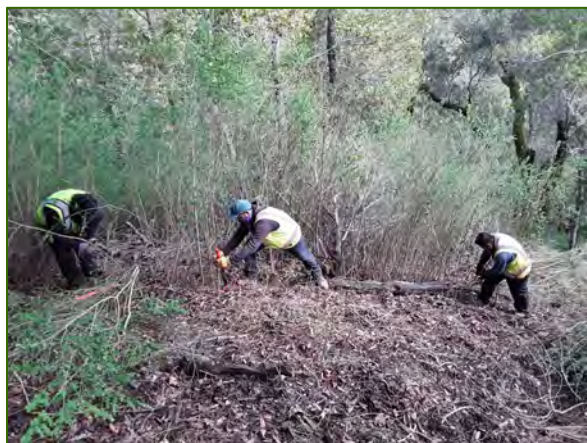
Photo 28: Concrete Pipe broom removal.
