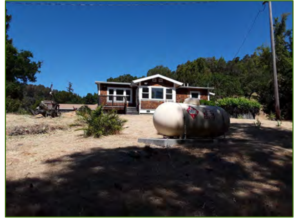
Photo 15: Porteous Residence After
