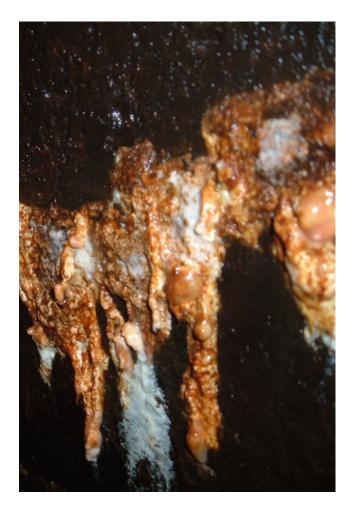
Evidence of groundwater infiltration, cracks, calcium deposits, and holes in the tunnel wall
