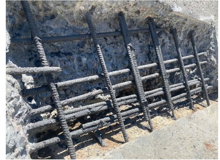
3. New #6, epoxy-coated rebar tied in, coated with corrosion inhibitor
