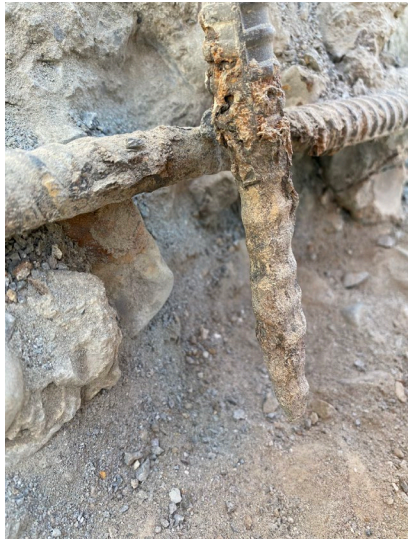
2. Corrosion removed
