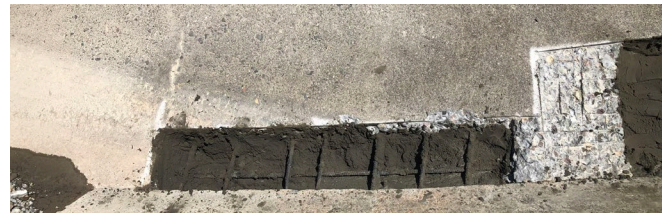
4. Low-shrink concrete placed in lifts
