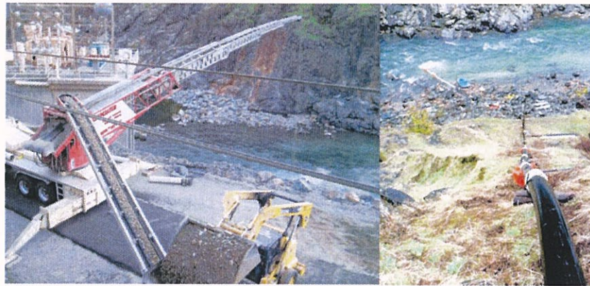
Figure 9 Gravel Augmentation Methods on the Yuba River
