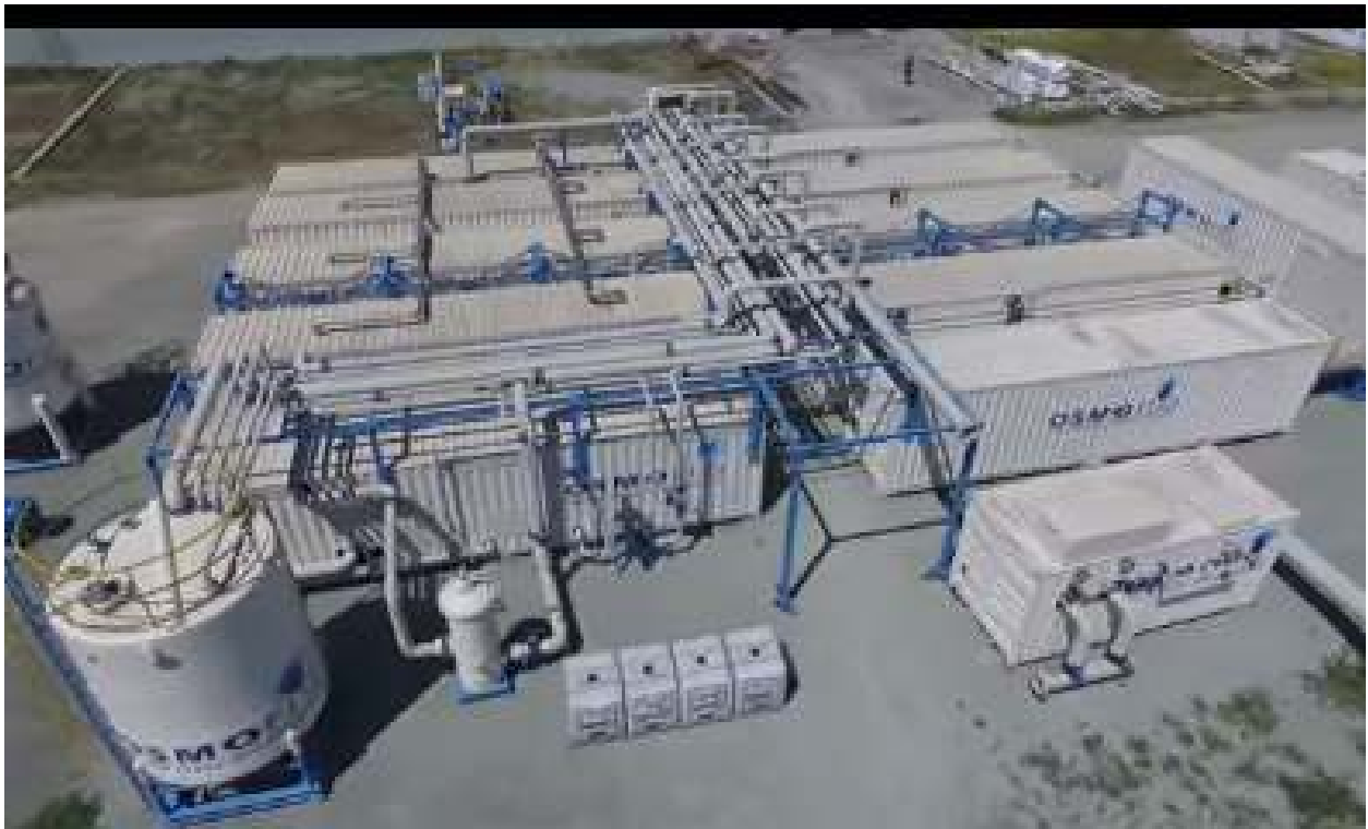
Figure 5: Osmoflo Containerized Seawater Desalination System (1.8 mgd)
