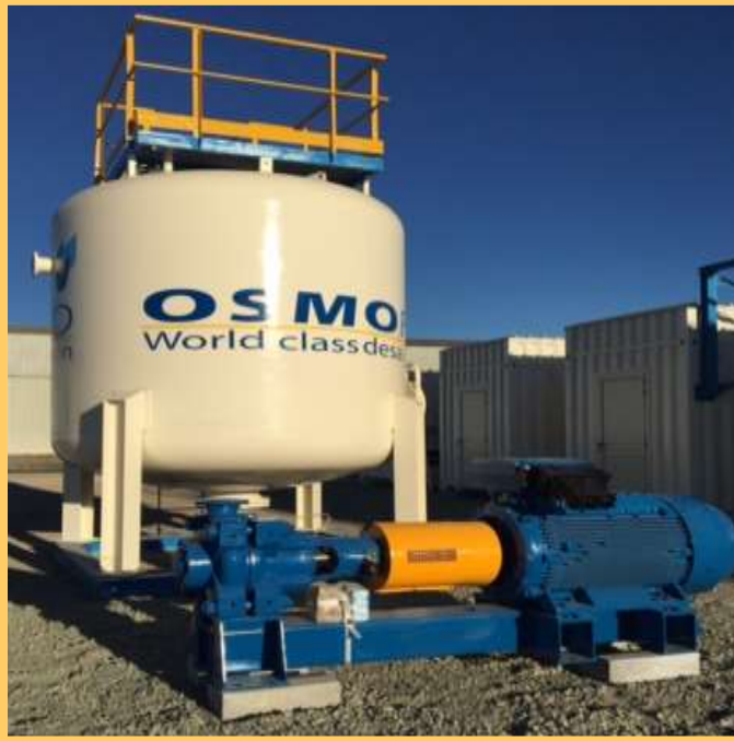
Calcite Filter & Product Transfer Pump
