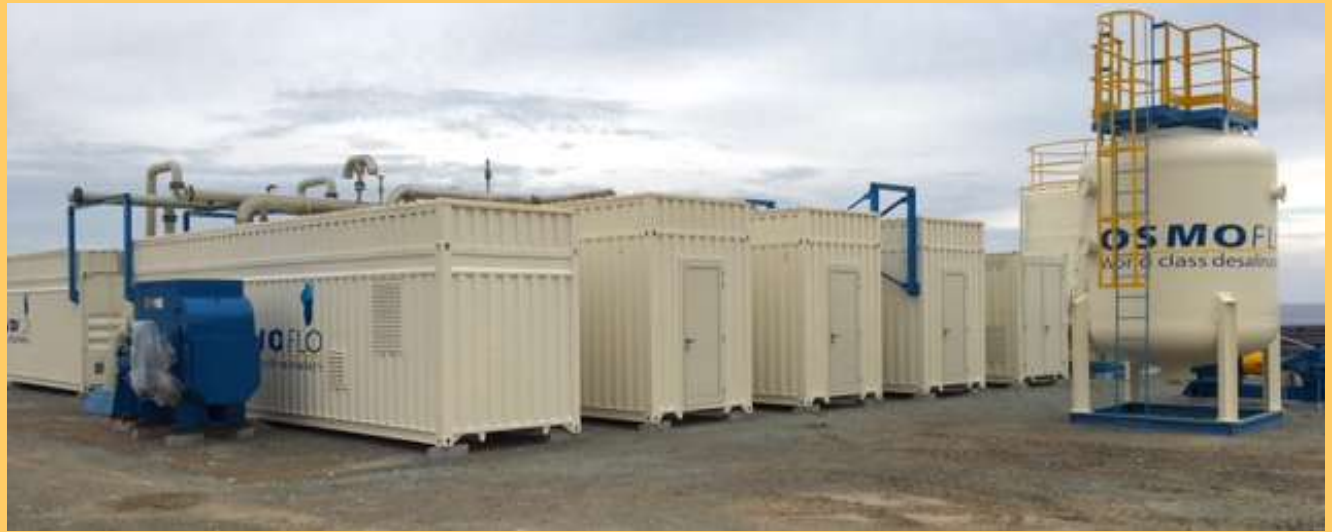
(R→L) HP Pump, LP&ERD Container, RO Containers, Calcite Filter
