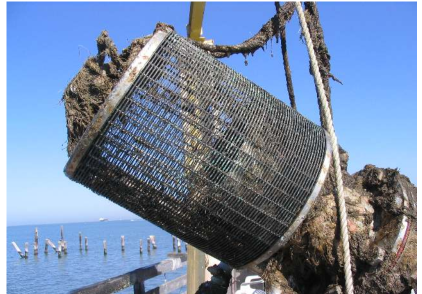
2006 Pilot Facility Intake Screen: 3/32-inch wedge-wire screen
