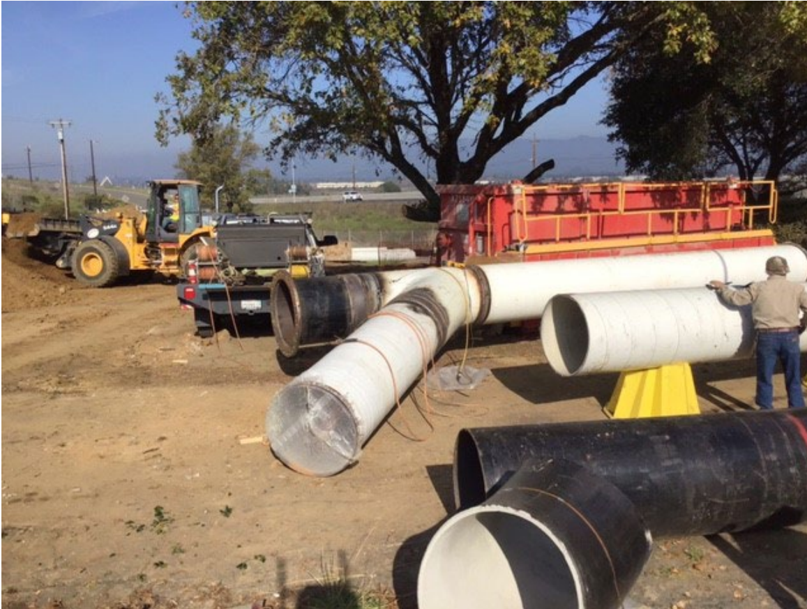
30" welded steel piping fabrication
