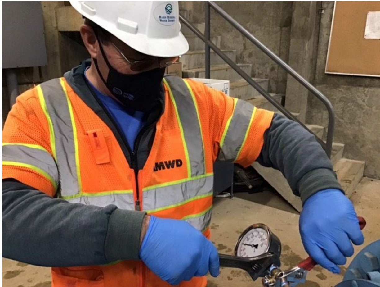
Marin Water's Rob Cuneo testing system pressure
