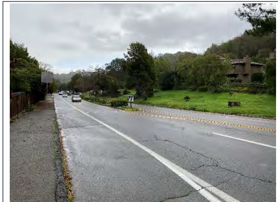
North San Pedro Road west of La Pasada Way has planted median islands that would restrict contractor access and work areas while maintaining acceptable circulation.
