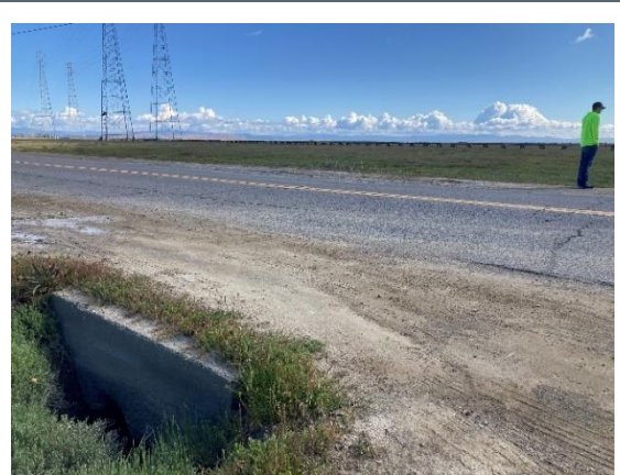
Culvert crossing is very shallow under North San Pedro Road.
