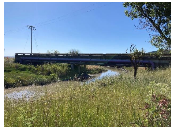
LGVSD has recycled water pipe (purple pipe) exiting their treatment facility. MMWD and North Marin Water District both use the facility's recycled water for irrigation.
