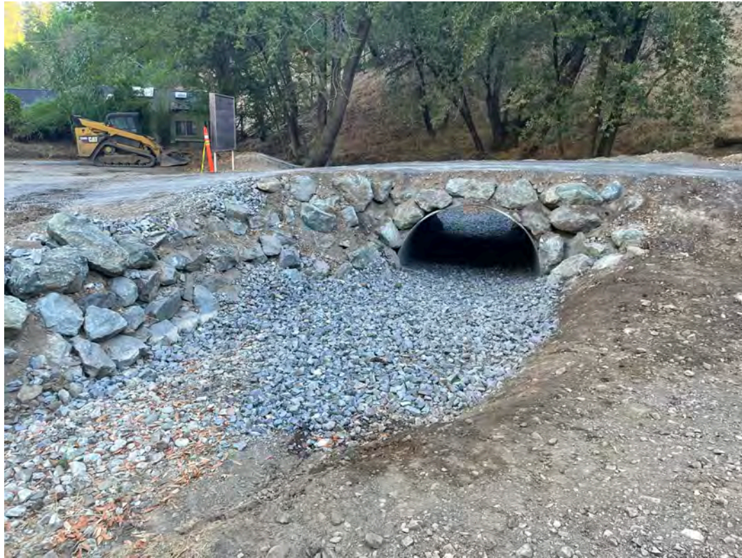
Marin Stables Culvert
