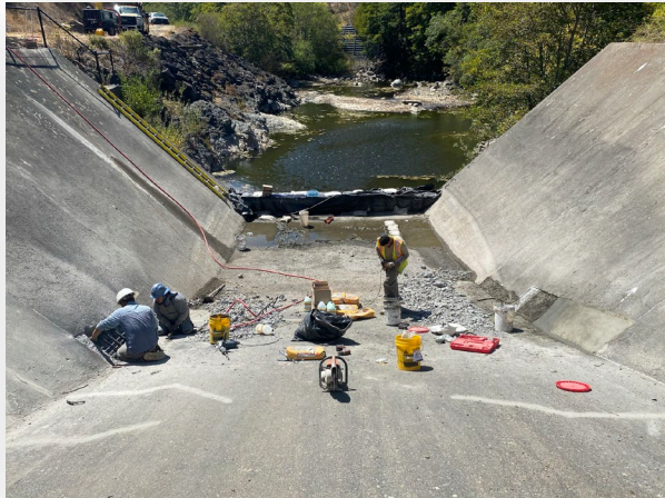
Non-structural spillway repair (Seeger Dam spillway, Nicasio Reservoir)
