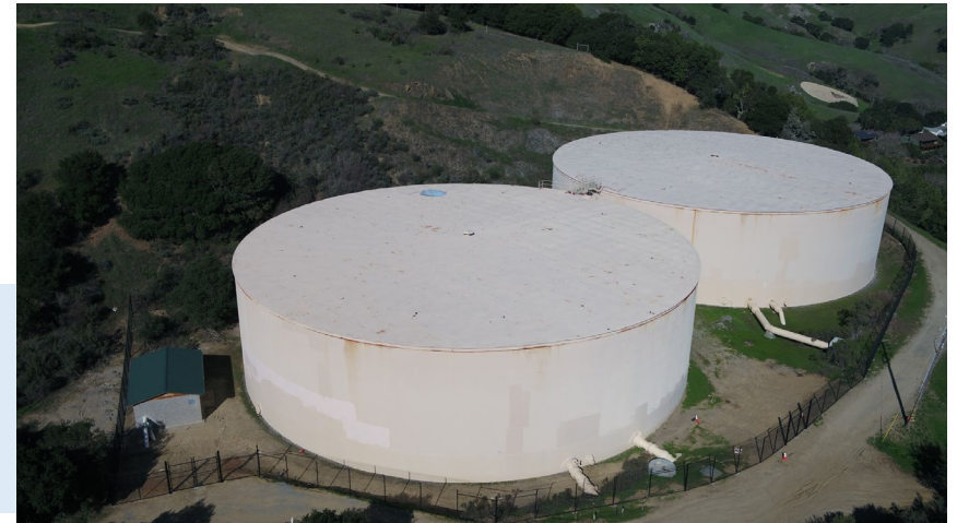
Smith Saddle Tanks Provide 10 MG of storage
