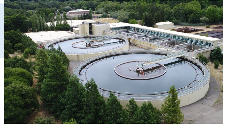
Existing San Geronimo Treatment Plant Clarifiers
