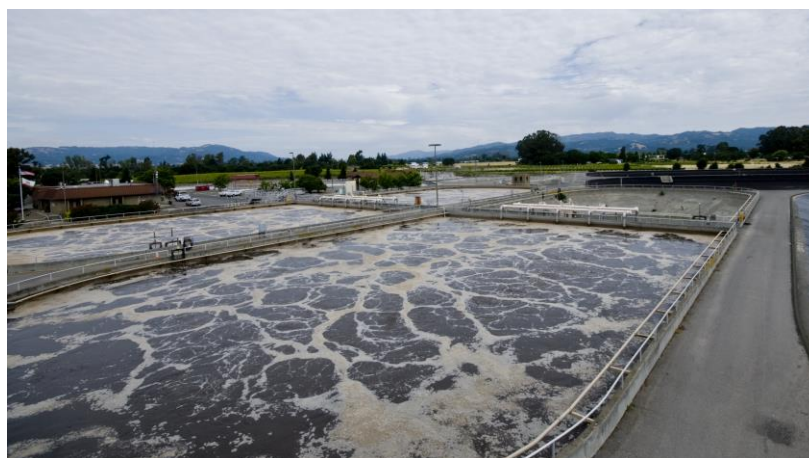
Wastewater treatment plant aeration basin.
