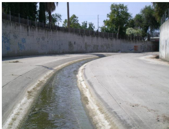
Multi-objective approaches to flood management aim to reduce the impacts of traditional channelized flood control infrastructure (above) by restoring creeks to provide both flood control and habitat benefits (below).
