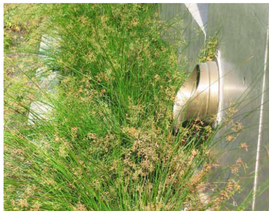
An interior roof drain discharges to a vegetated swale in Emeryville, CA. This is an example of an “approved alternate location” for stormwater discharge.
