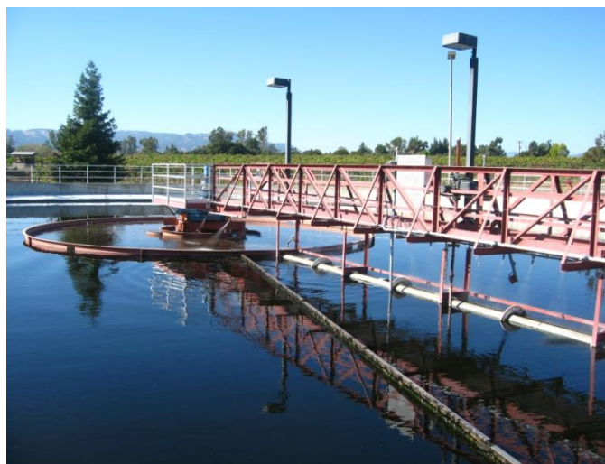
Sonoma Valley Wastewater Treatment Plant, Clarifier
