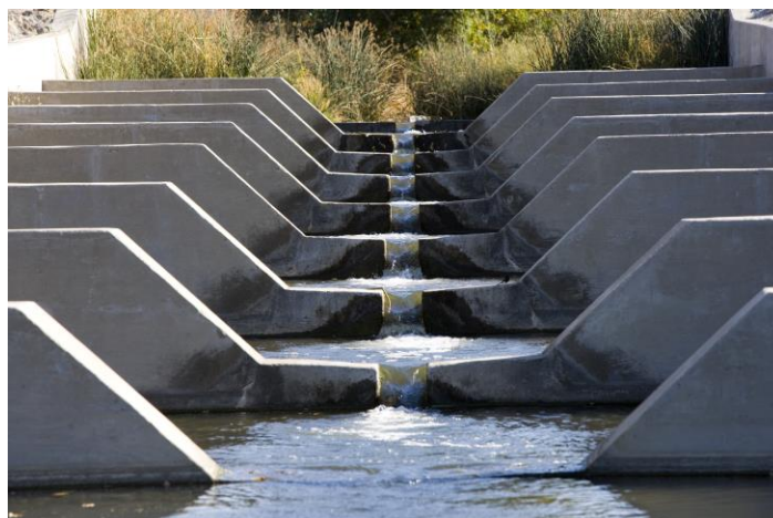
An example of a fish ladder installed as to aid fish passage on a Bay Area stream.
