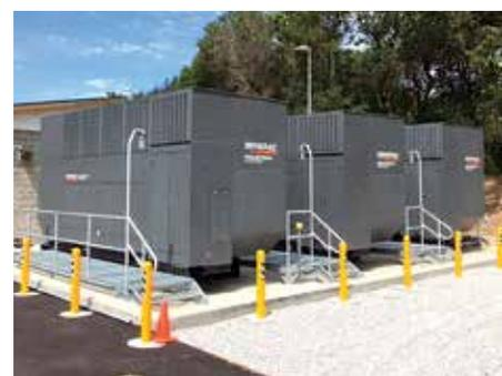
Three permanent emergency generators were installed at the San Geronimo Treatment Plant in 2022 to ensure continued water service for customers in the event of a power outage. The rate proposal will allow for additional water system reliability enhancements.
