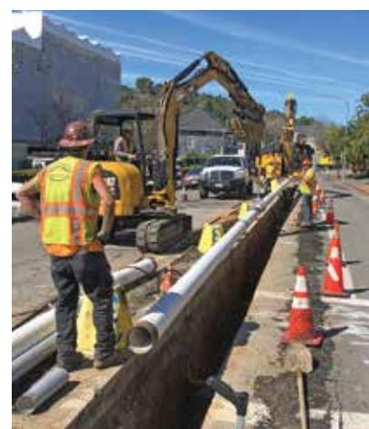
A 2022 pipeline replacement project on Third Street in San Rafael replaced 6,570-feet of 95-year-old cast iron pipe with new welded steel pipe. The proposed rate adjustment will increase the amount of aging pipeline Marin Water is able to replace per year.
