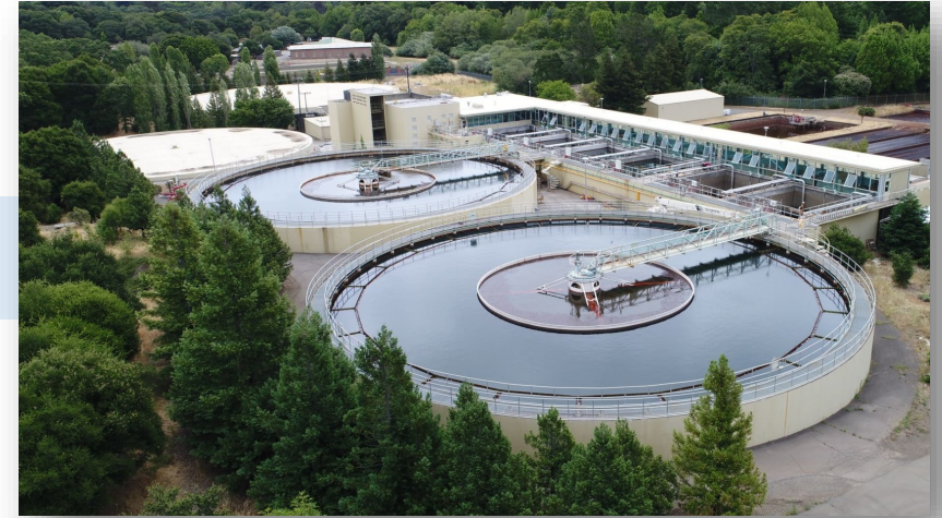
Existing San Geronimo Treatment Plant Clarifiers
