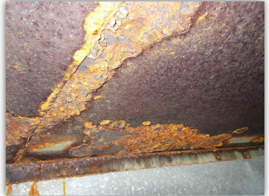
Current condition (interior)
