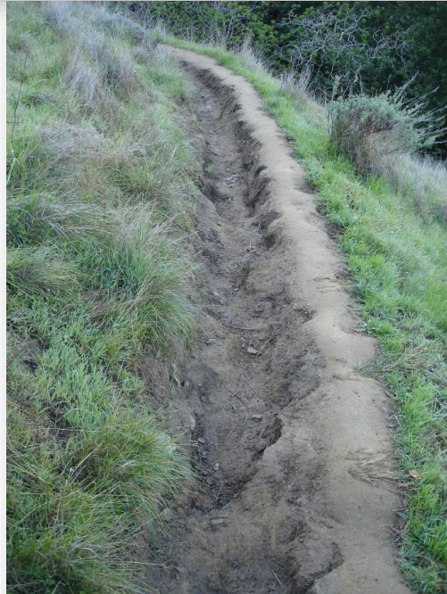
Left: Culvert Replacement (Top); Trail Restoration (Bottom);
