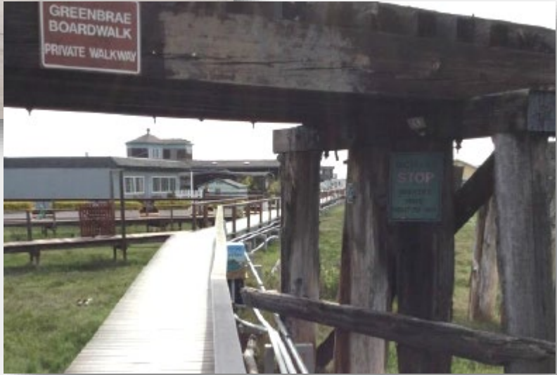
Greenbrae Boardwalk Pipeline Replacement
