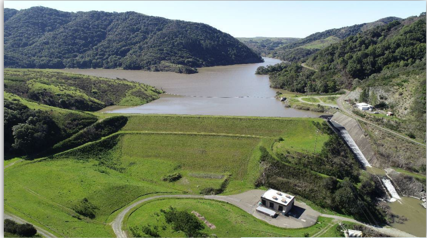
Soulajule Dam & Pump Station
