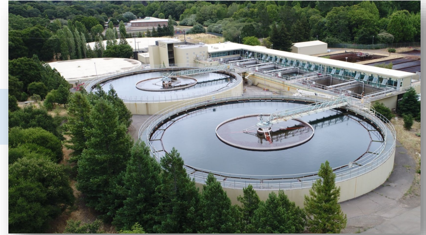
Existing San Geronimo Treatment Plant Clarifiers
