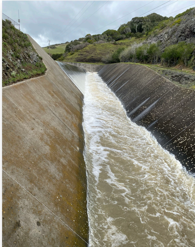
Spillway Repairs (Seeger Dam)
