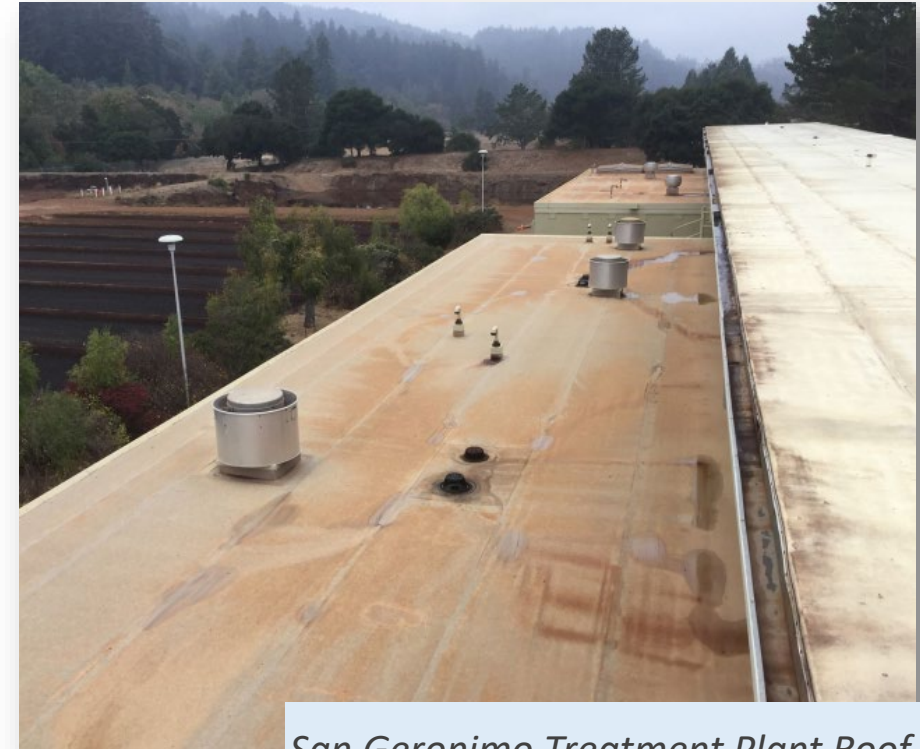
San Geronimo Treatment Plant Roof
