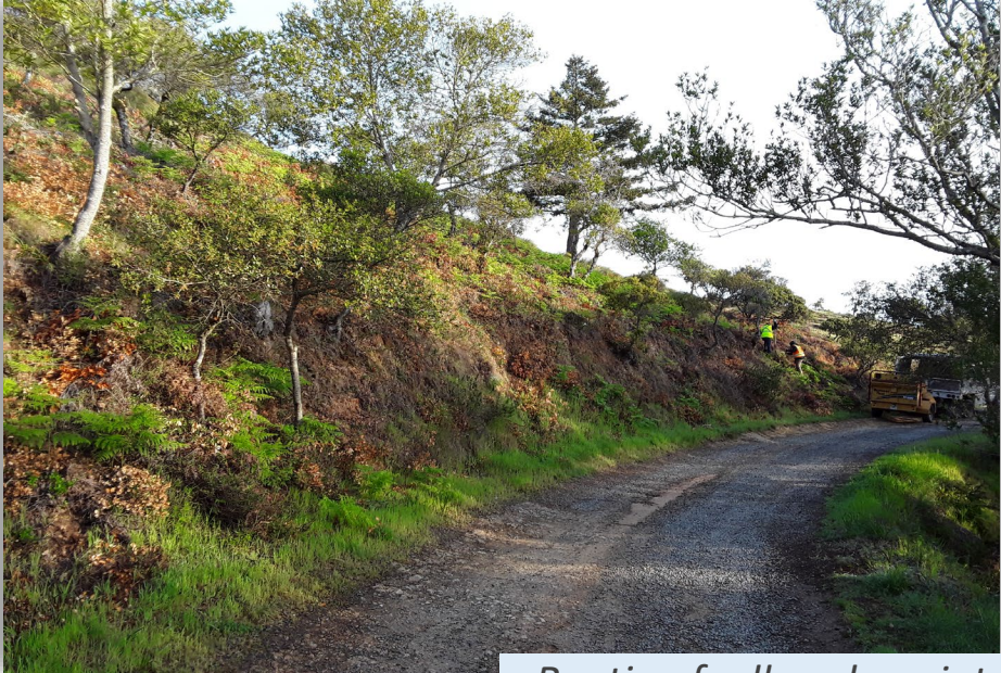
Routine fuelbreak maintenance along Lower Railroad Grade
