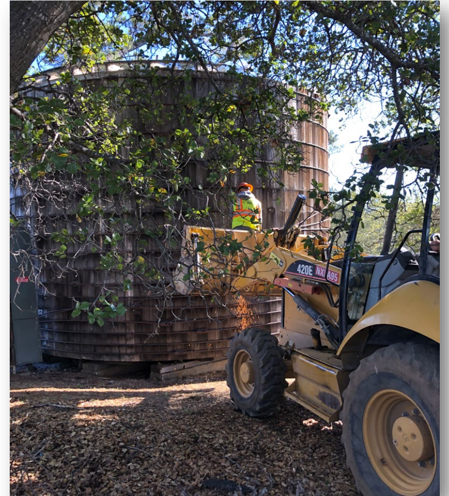
Courtright Tank System Improvement (project completed October 2022)
