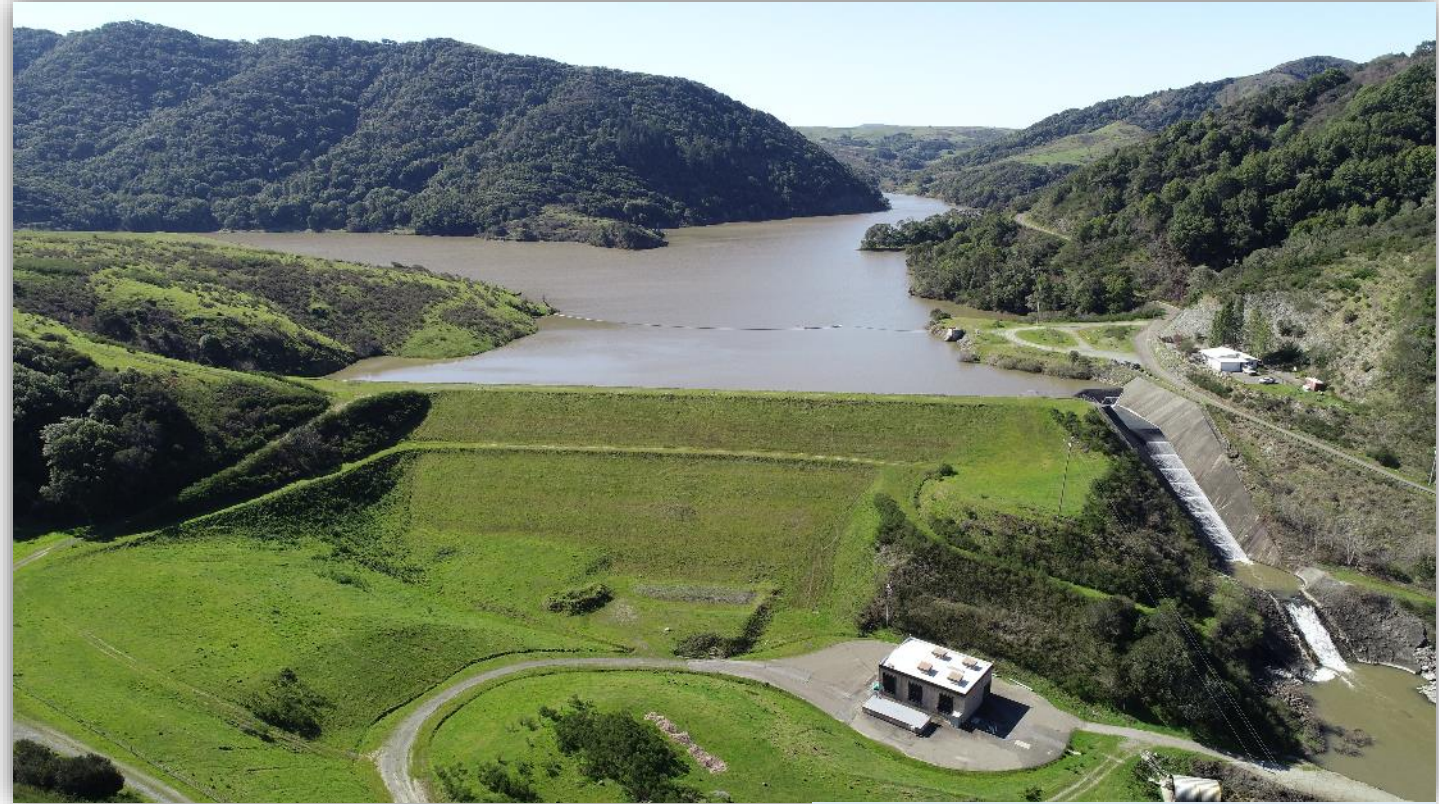
Soulajule Dam & Pump Station
