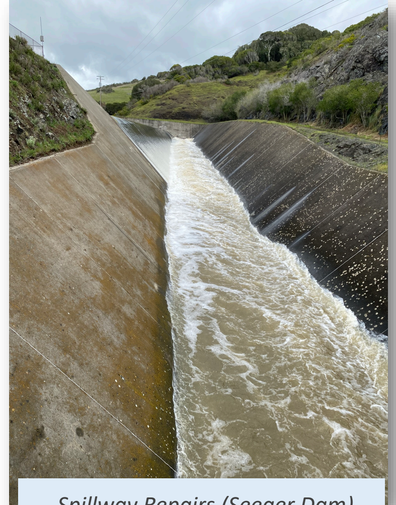
Spillway Repairs (Seeger Dam)
