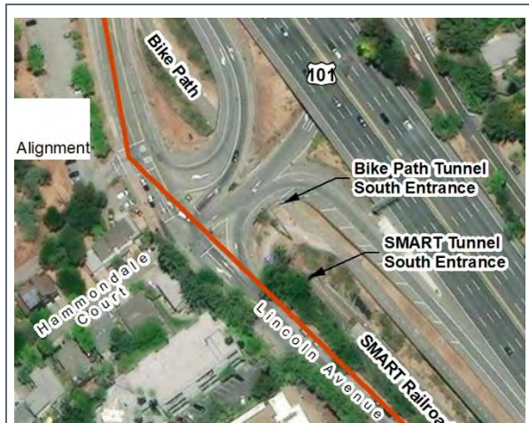
Aerial view of SMART Tunnel, bike path tunnel, US 101 on and off-ramps at intersection of Lincoln Avenue and Hammondale Court.
