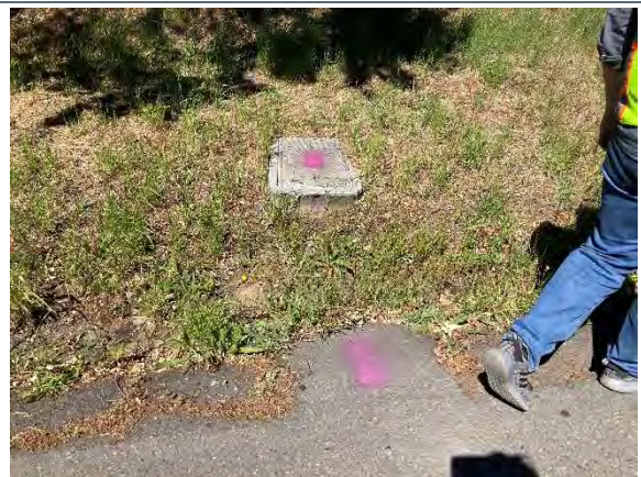
South Alignment's connection to the existing recycled water system on the north side of Merrydale Road south of North San Pedro Road.
