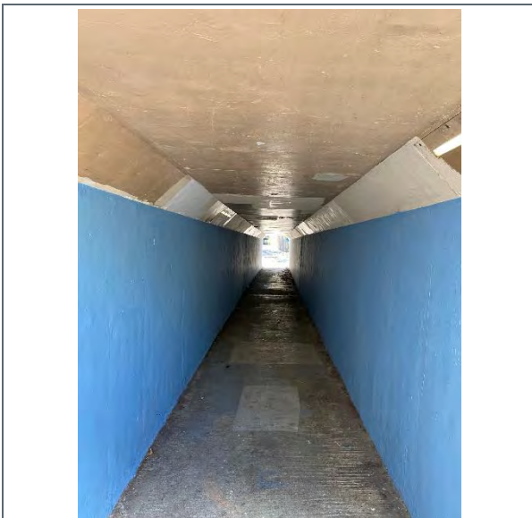
San Pedro Elementary School underground pedestrian crossing.
