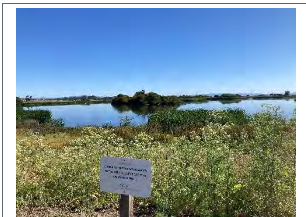
LGVSD has three reclamation ponds that are used primarily as recycled water storage facilities.
