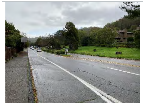
North San Pedro Road west of La Pasada Way has planted median islands that would restrict contractor access and work areas while maintaining acceptable circulation.
