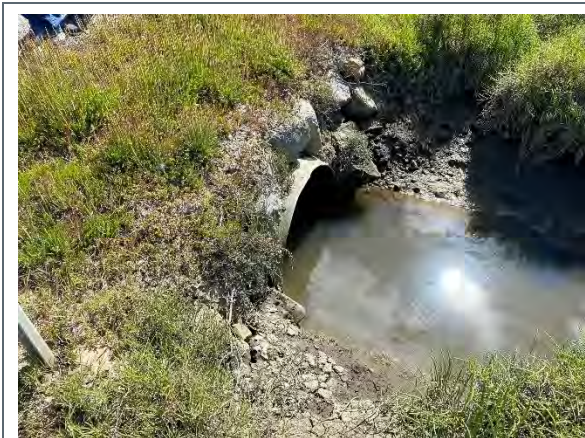
Culvert crossing under North San Pedro Road.
