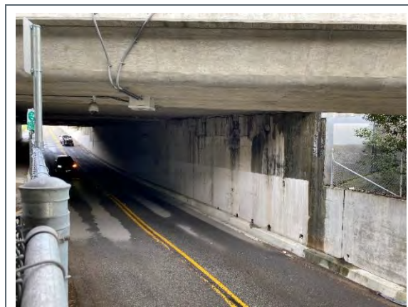
Looking southwest along the Linden Lane undercrossing.
