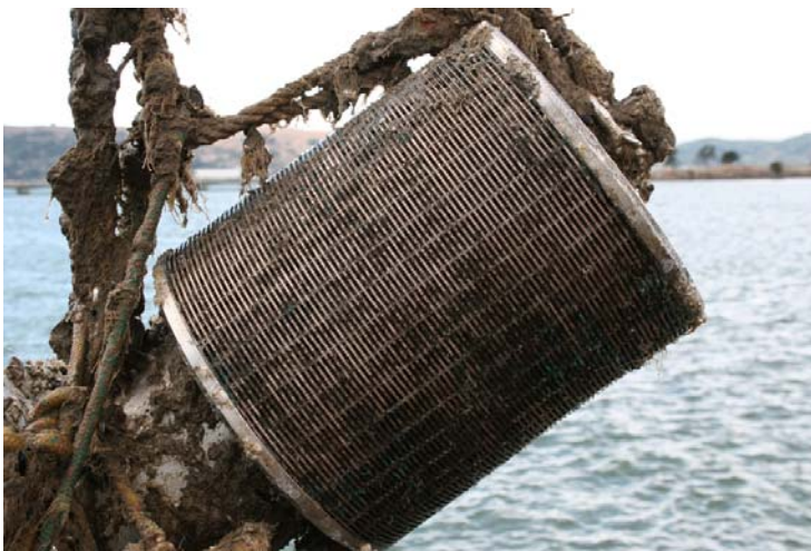
Intake Screen after manual cleaning 8 August 2005
