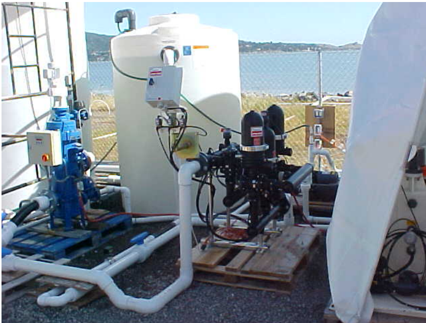
Bollfilter strainer on the left and Arkal Strainer on the right
